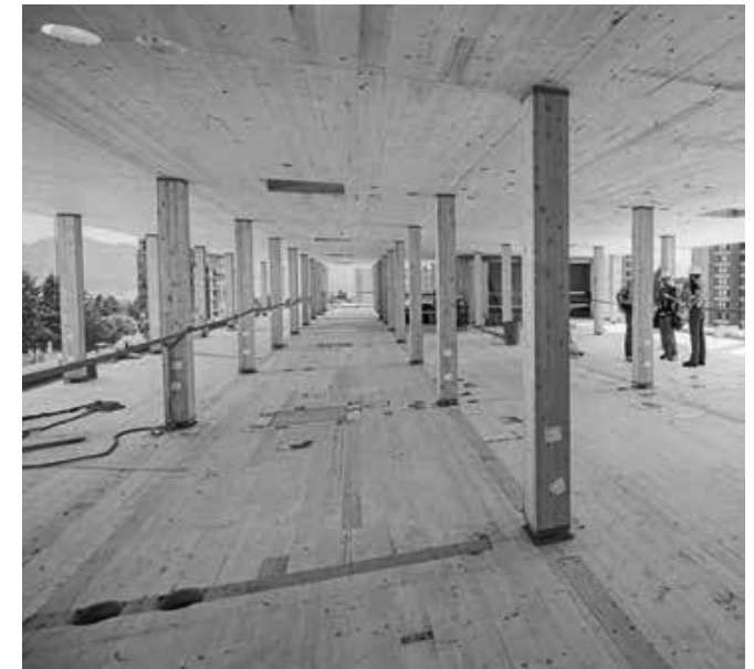
Figure 3.3: Columns i.c.w. CLT floors
