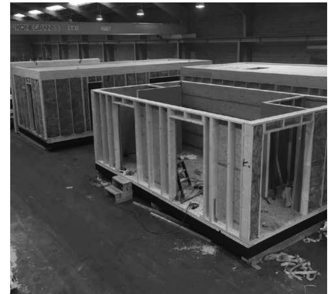
Figure 7.3: Prefabricated modules made of timber framing
