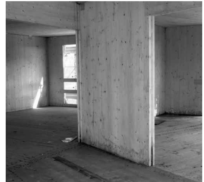
Figure 6.3: CLT walls and floors
