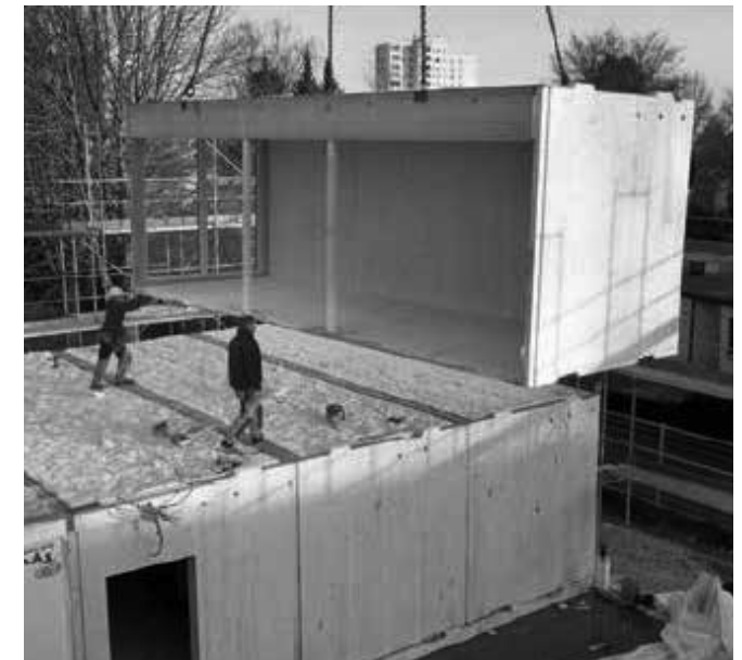
Figure 8.3: Ready made modules assembly
