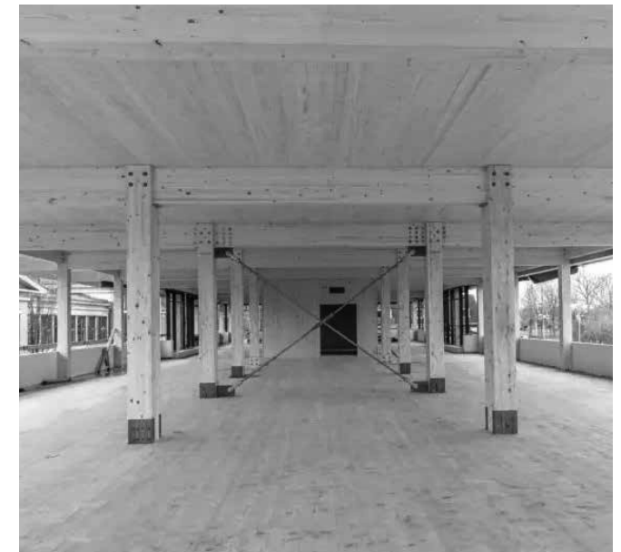
Figure 2.3: Column/beam construction i.c.w. CLT floors
