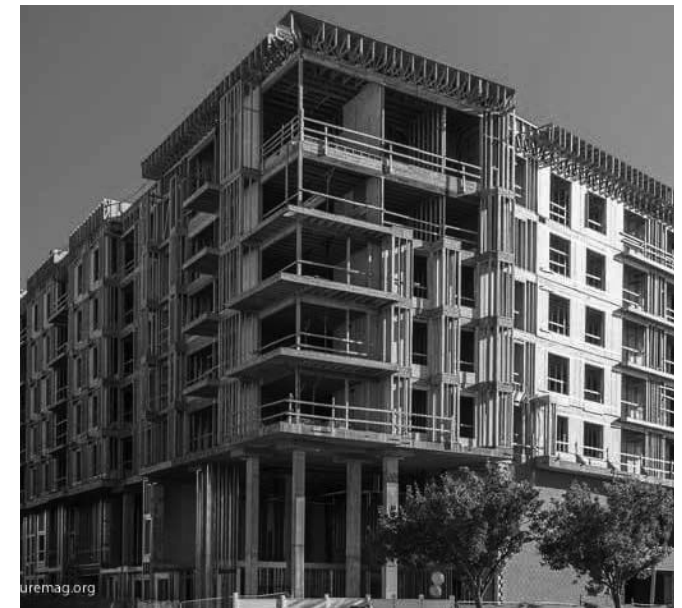
Figure 4.3: Timber frame construction
