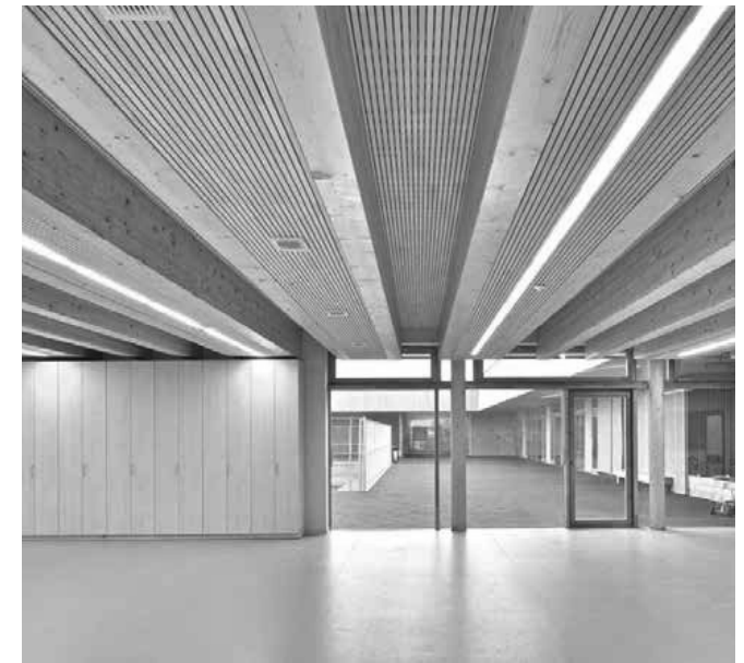
Figure 5.3: Mass timber walls i.c.w. laminated beams
