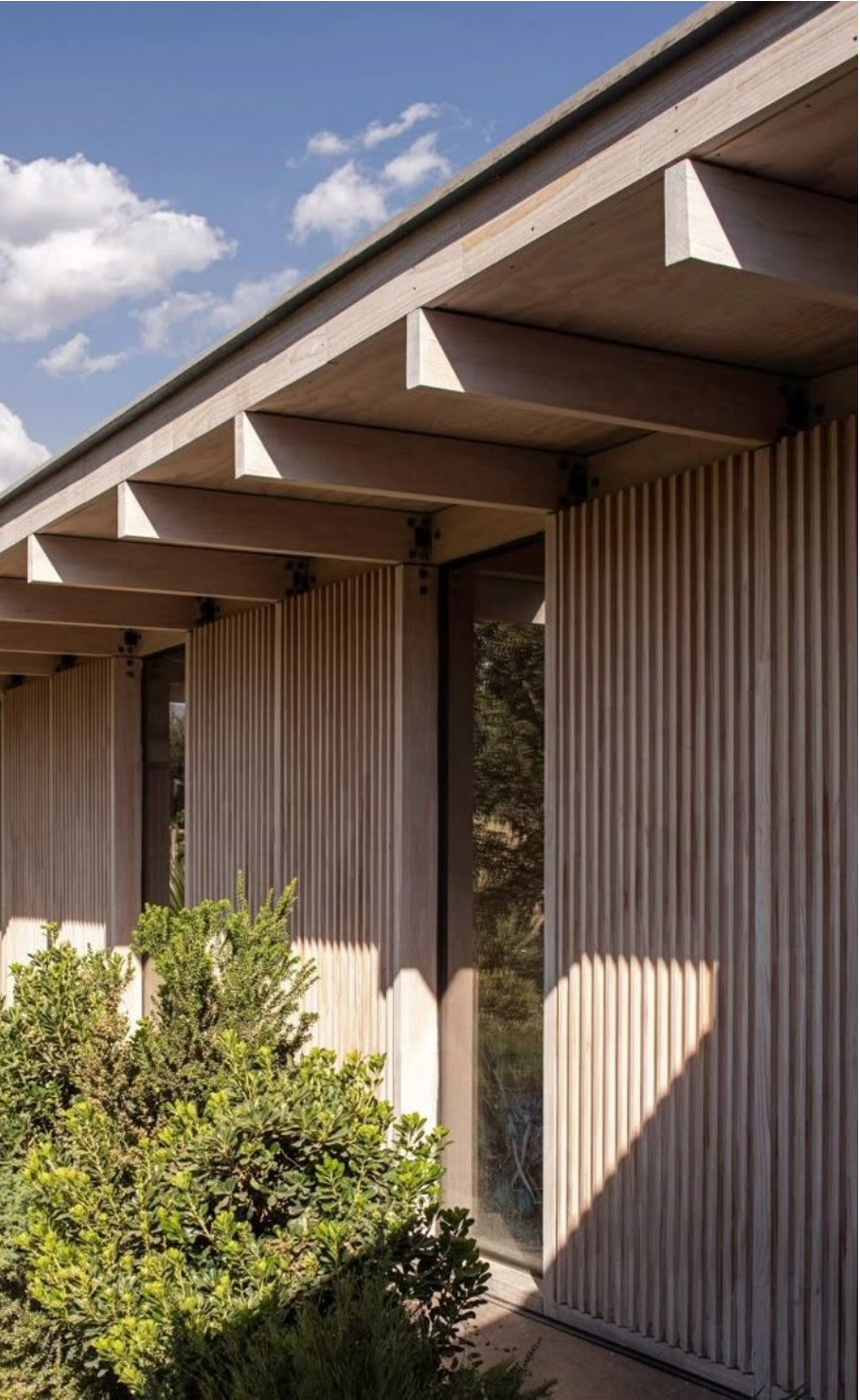
MasFernandez Arquitectura tops Chilean home
