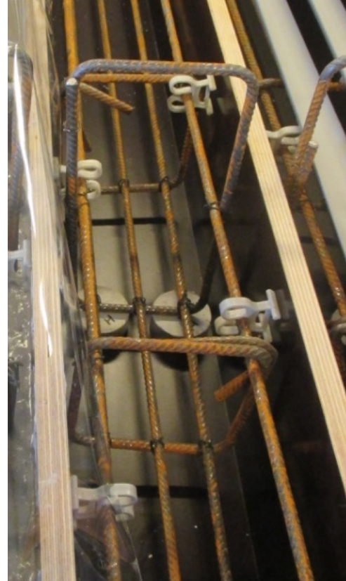
Figure 32 Rebar cage in the mould with spacers
