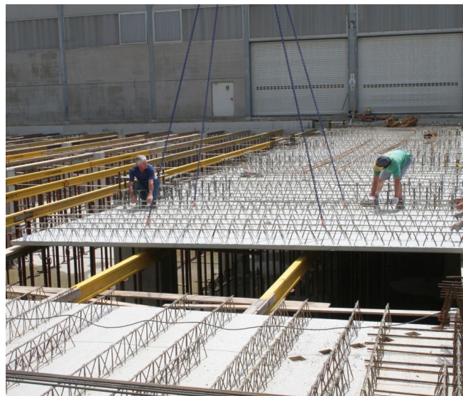
Figure 5 Lattice girder floor
