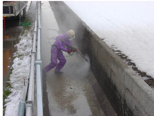
(b) Surface Preparation
