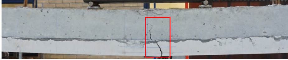
Figure 74 Beam with SHCC+SH layer of 70 mm, after failure, under the load of 40 kN
