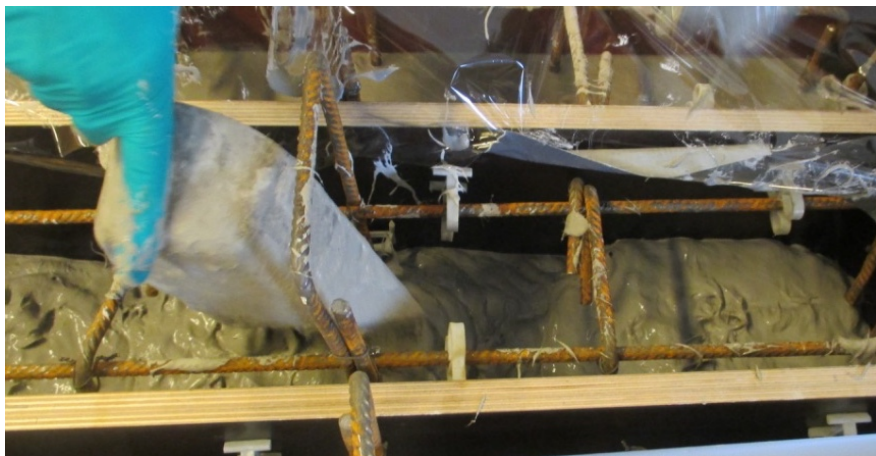
Figure 34 Spoons used in casting SHCC layer
