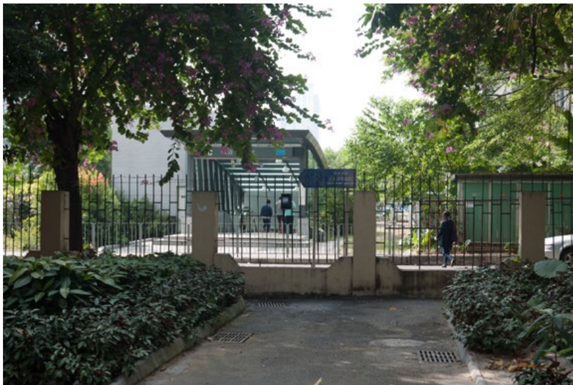
Lack of connection
