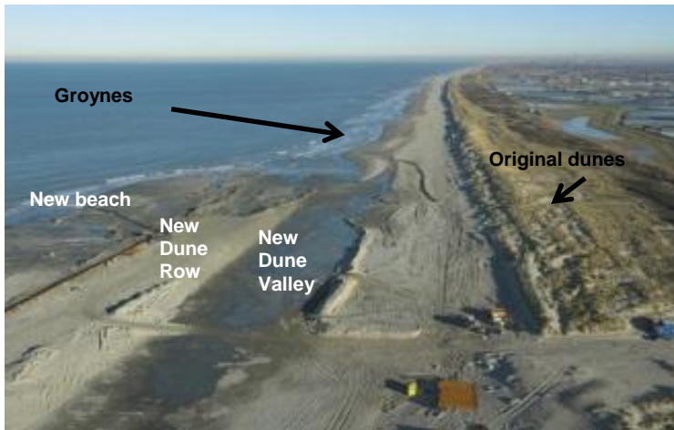
Figure 2: Aerial photograph of the Vlughtenburg field site during construction of the nourishment in 2009. Original beach and vegetated dunes visible on the left. (source: www.delflandsekust.nl )
