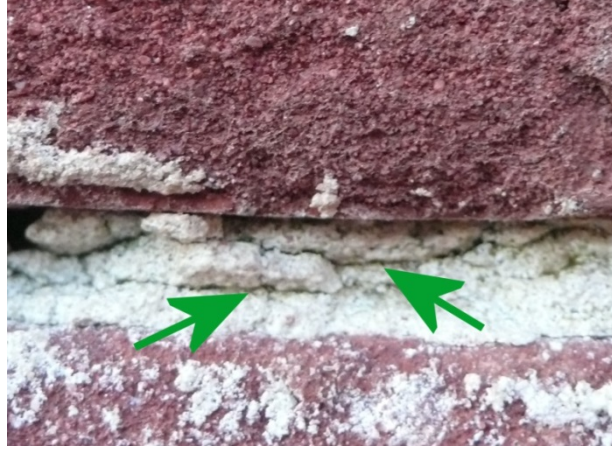
Figure 4. Frost damage in an uncarbonated air lime mortar due to an application of the mortar too late in the season (Brussels, Belgium)
