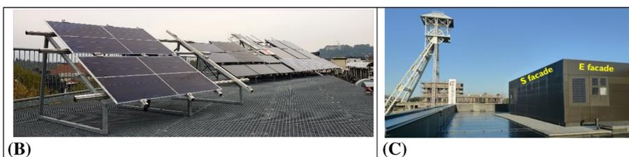
**FIGURE 16** (A) List of sites for outdoor monitoring of BAPV (red) and BIPV (blue) modules. (B) BAPV monitoring site at University of Ljubljana (UL) in Slovenia (azimuth: south, tilt:  $30^\circ$ ). (C) BIPV monitoring site at imec in Genk in Belgium (azimuth: south and east, tilt:  $90^\circ$ ) [Colour figure can be viewed at [wileyonlinelibrary.com](http://wileyonlinelibrary.com)]
