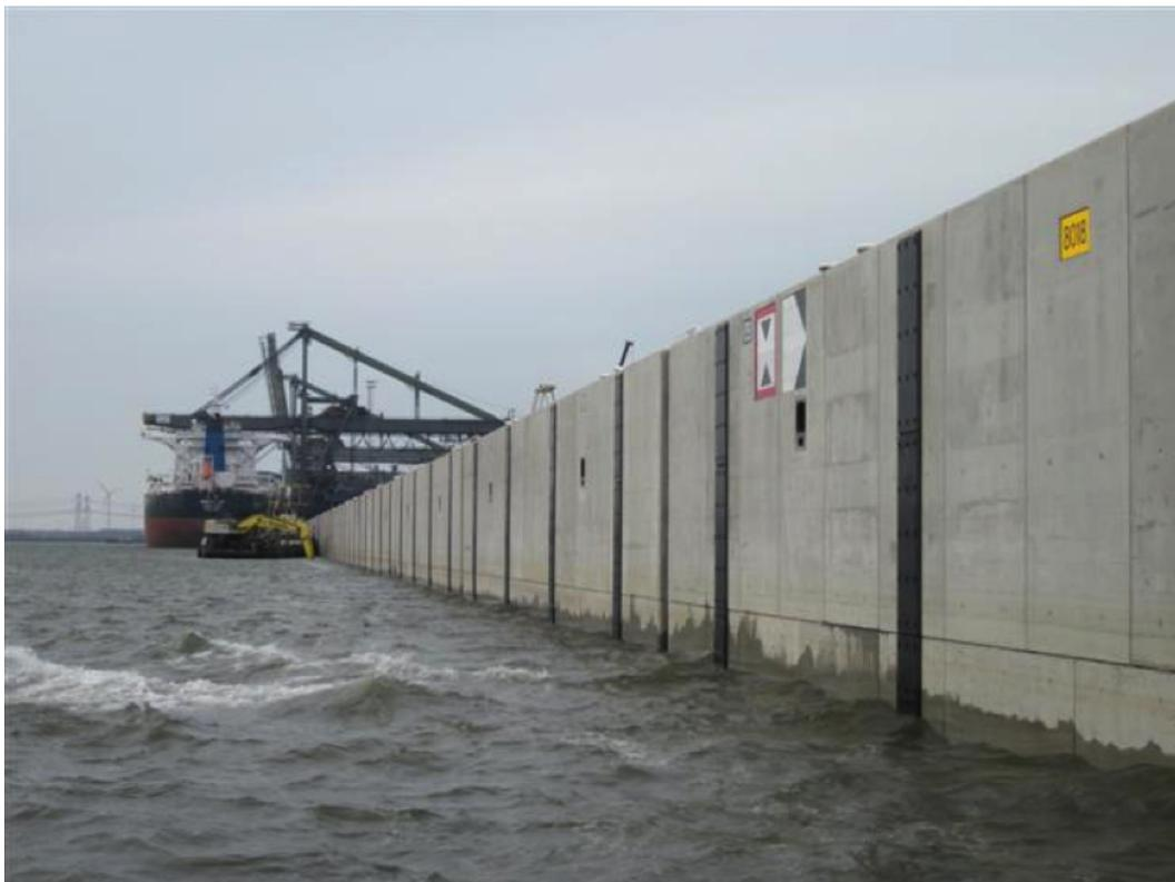
FIGURE 3.6: Fendering of SFRHPC, EMO coal quay Rotterdam
