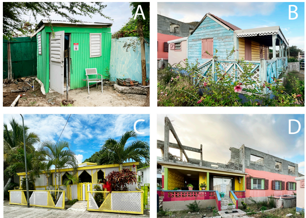
Figure 3. Impressions of different types of self-organized housing on St. Martin. (A) small housing unit at Pond Island using temporary materials; (B) light balloon-frame timber house with a porch and concrete extension in the back; (C) pre-fabricated concrete house with porch built as an extension; (D) house built with concrete blocks with an unfinished upper floor. Source: authors.
