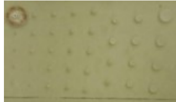
(b) Image of the damaged panel. The burnt epoxy can be seen in the image caused by the spindle when it crashed into the panel.
