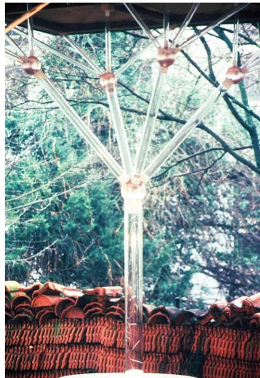
Figure 20 Tubular extruded glass column tree structure in Aachen, Germany for (Knaack, 1998)
