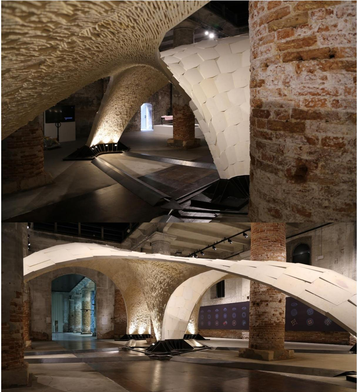
*Figure 143 The Armadillo Vault, showing a fixed support and tension-based foundation creating a compression ring effect (Frearson, 2017).*
