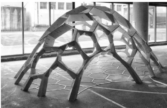
Figure 72 The Concrete Grid shell (Pedersen et al., 2014)
