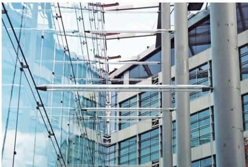
Figure 19 Tower Place in London. Pre-stressed structural glass tubes (Bhatia, 2019)
