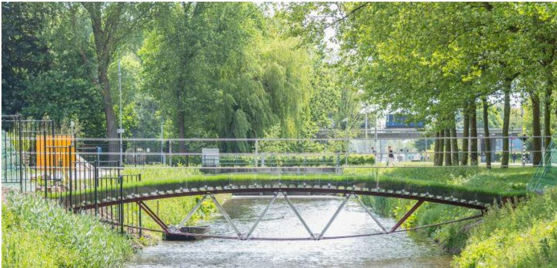
Figure 22 The glass truss bridge (Snijder et al., 2018).
