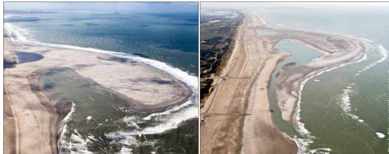
The sand engine after construction on August 9, 2011 (left) and the condition on January 10, 2012.
