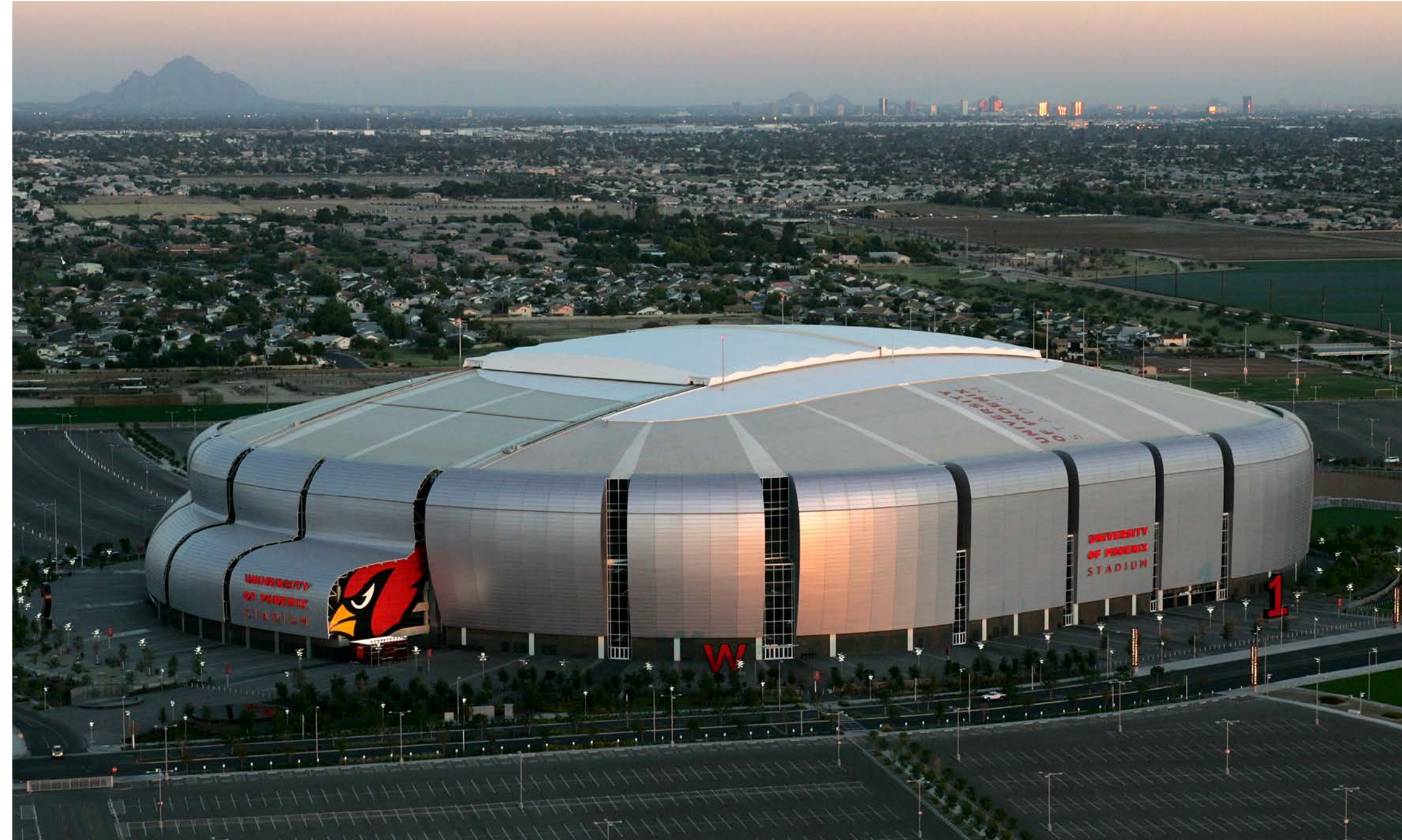
UNIVERSITY OF PHOENIX STADIUM (2006) HOUSTON, TEXAS DESIGN: EISENMAN ARCHITECTS, POPULOUS
