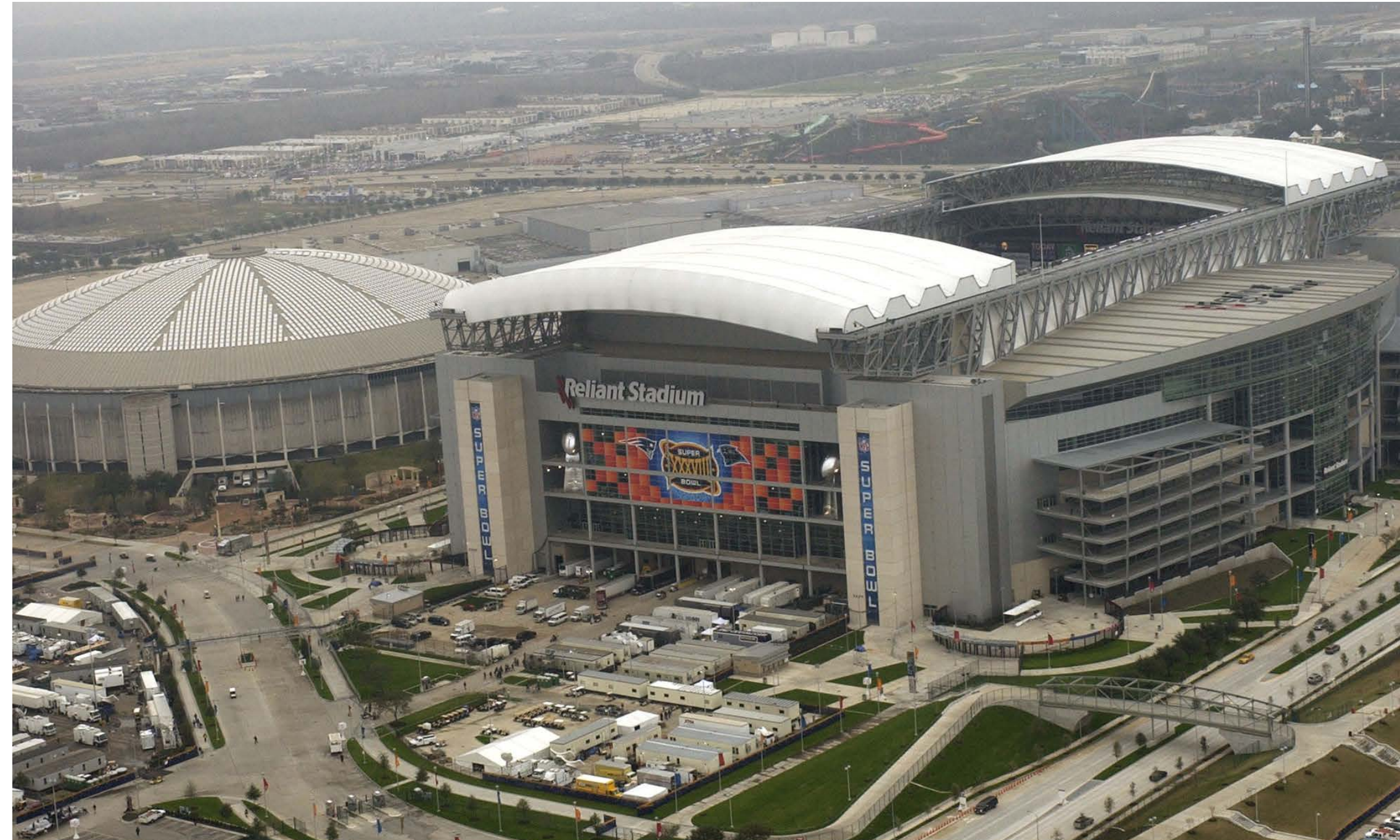
NRG STADIUM (2002) HOUSTON, TEXAS ARCHITECT: POPULOUS
