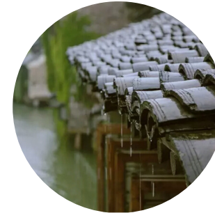
Roof tiles show direction for rain water to drop.
