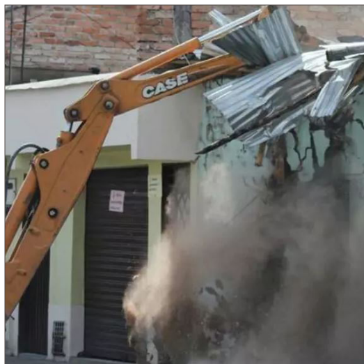
Fig. 2.2.3: Medellín, demolition of illegal buildings
