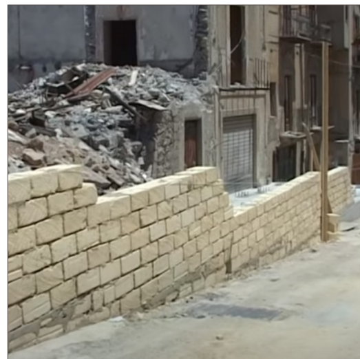
Fig. 2.2.4: Favara, tuff wall
