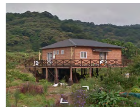
Stilt house in high flood risk area
