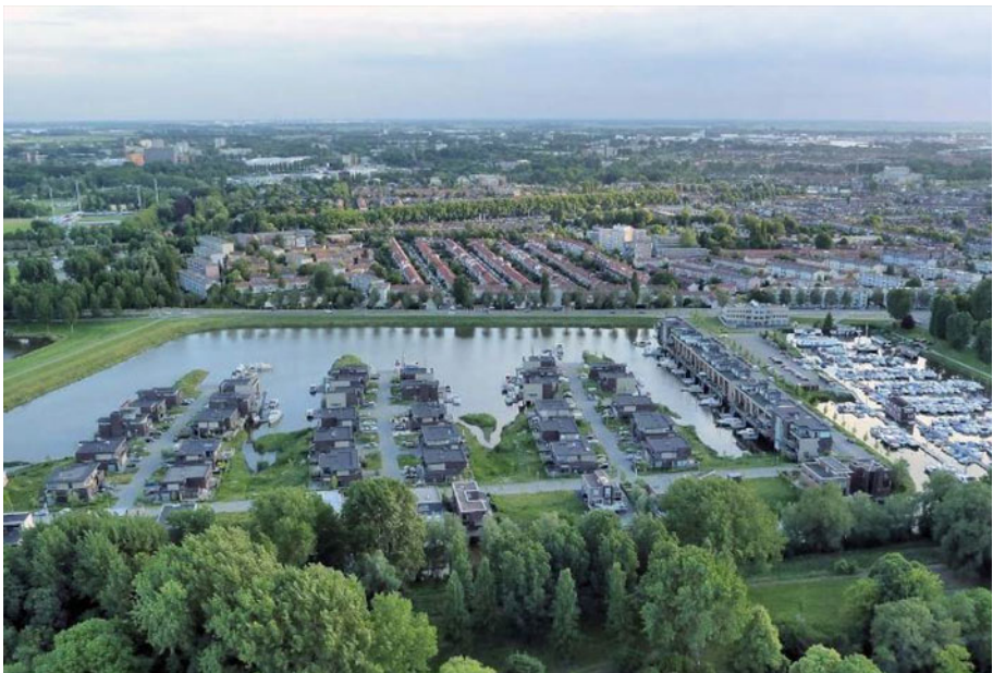
Fig. 2 Full-scale in situ experiment to explore the Multi-Level Safety approach in the City of Dordrecht within the Delta Programme (courtesy City of Dordrecht)
