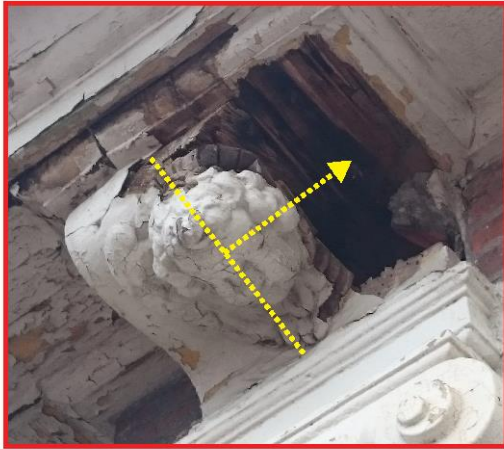
Extrapolation using the symmetry of the test candidate relief
