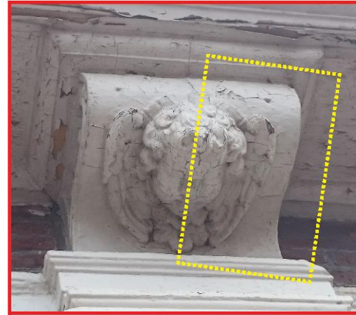
Extrapolation using existing geometry from undamaged relief
