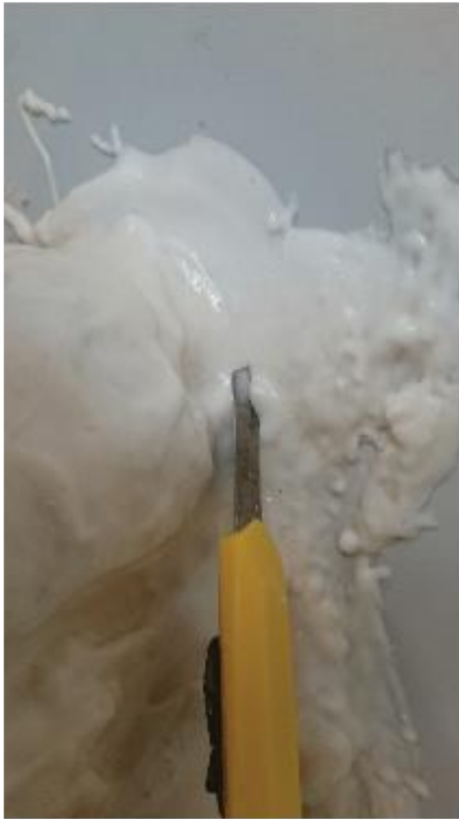
Overflow cut off
