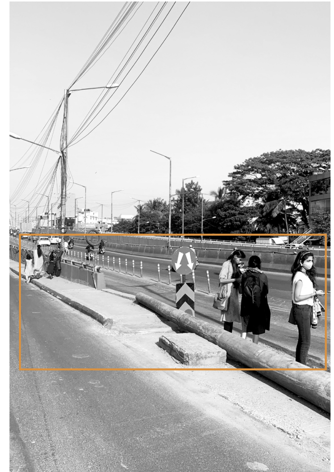
Img 23: Unsafe pedestrian infrastructure Source: Author
