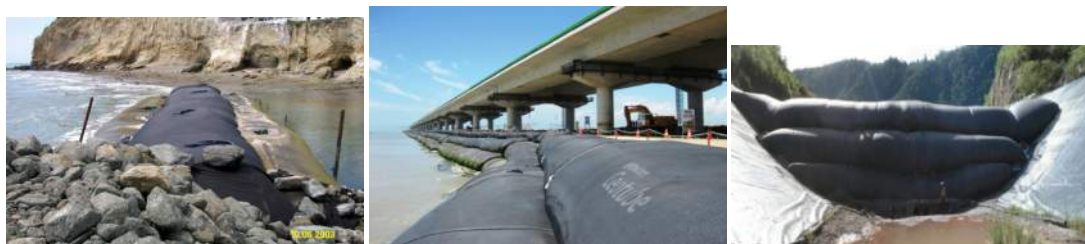
Figure 10.17: Staked tube application [?] ]
