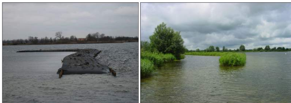
Figure 10.15: Geotextile Tubes for shoreline protection with vegetation by tencate [? ]
