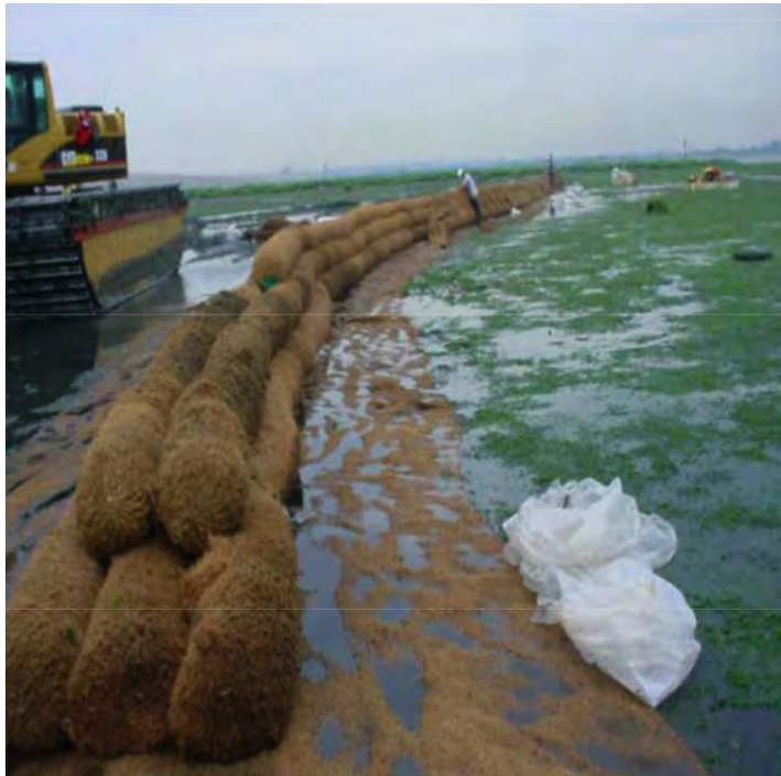
Figure 10.11: Elders point East is restored with coir log (USACE [63])
