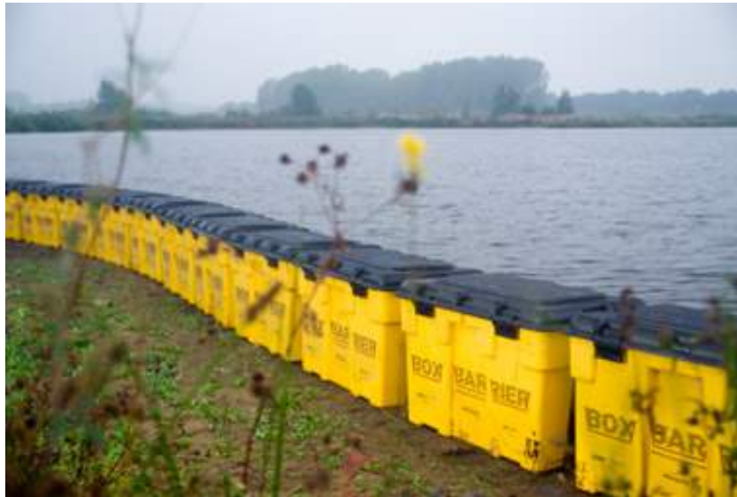
Figure 6.3: An example of a BoxBarrier application; box elements are filled by water and connected by joint elements
