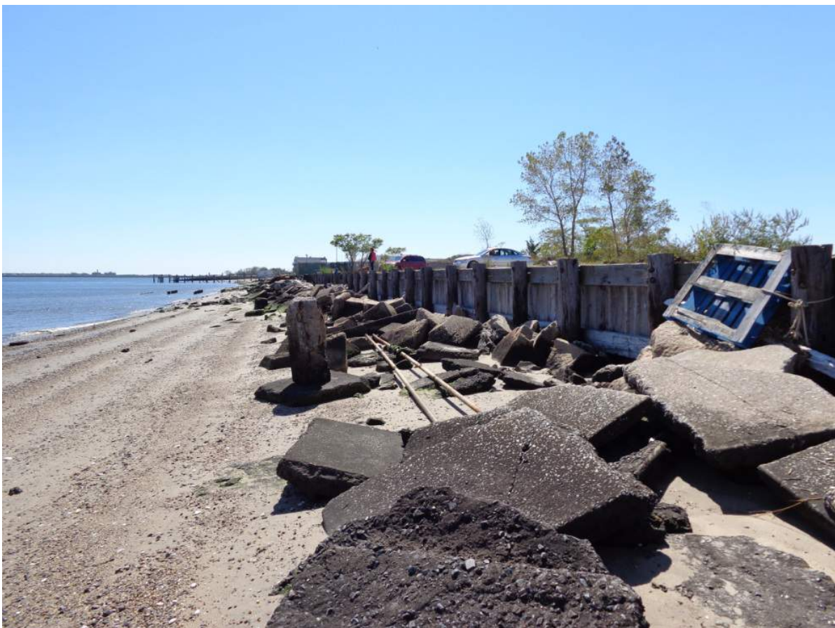
Figure 7.15: Revetments at Floyd Bennett Field
