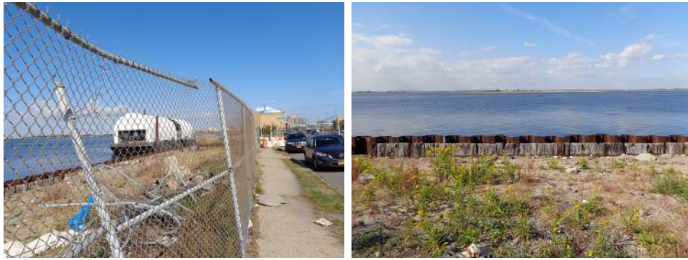
Figure 5.7: Sheetpiled bank and available space adjacent to Beach Channel Drive
