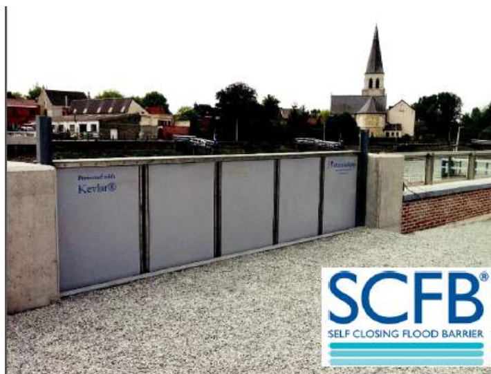
Figure 6.5: SCFB barrier in position, Schelle Belle Belgium
