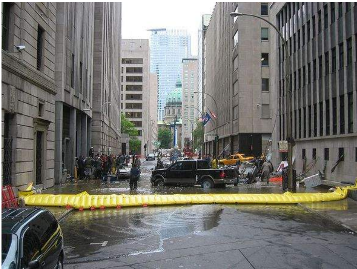
Figure 6.2: The Watergate system protecting the National Archives in Washington DC
