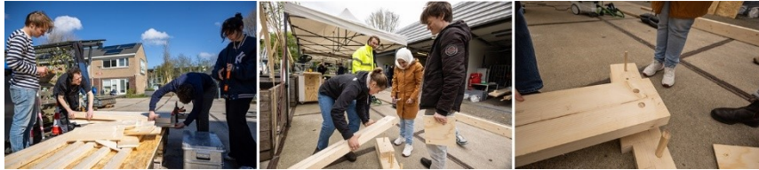
Figure 2 Students of CPD experimented with developing a DLT structure. After cutting all wooden elements in the desired dimensions, the planks were assembled using wooden dowels.
