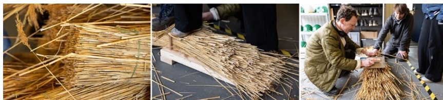
Figure 3 Thatching is one of the emerging trends not only as a finishing layer for roofs, but also for cladding. Students of CPD experimented with layering the reed batches on a façade and tried to perform thatching rituals to achieve the desired texture.
