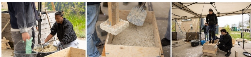
Figure 5 Hempcrete construction through the stages of mixing, ramming and even 'jumping' to achieve compaction during the CPD course.
