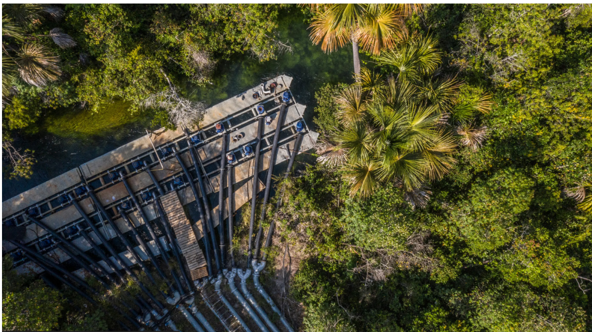
Image 3.2 Pumps taking water from the Arrojado River to the irrigation system of Rio Claro farm in
