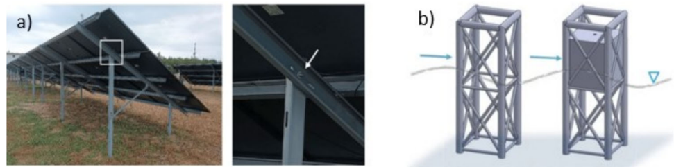
Fig. 8 Examples of steel applications in energy structures: a a substructure for photovoltaic panels made of thin-walled cross-sections with typical bolt connectors (Mrówczyński et al. 2022); b a jacket-type structure installed with OWC converter (Zhang et al. 2020a, b)
