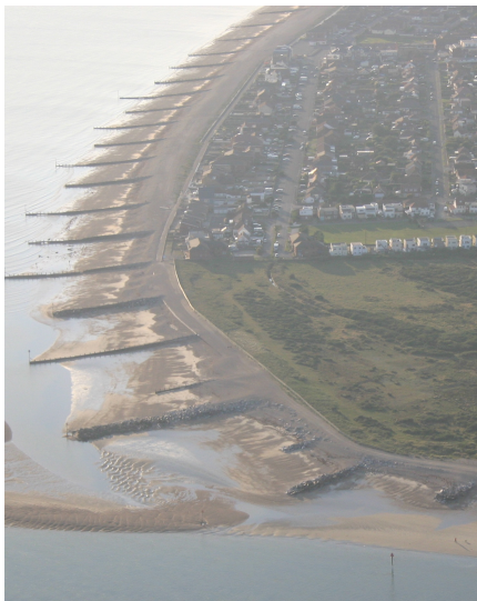
Figure 1.1: A groin system in Hayling, UK, as a coastal protection system (Maritimejournal, 2014). Sediment accumulates in the groin fields.
