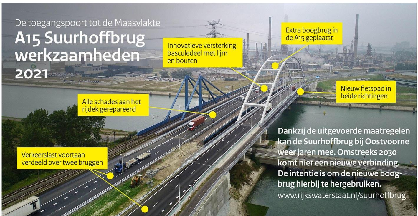
**Figure 41: Overview strengthening interventions Suurhoff bridge (Rijkswaterstaat, 2021)**
