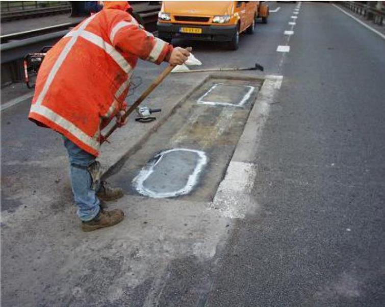
**Figure 23: Two covering plates installed during a reparation (van Dooren, 2018)**
