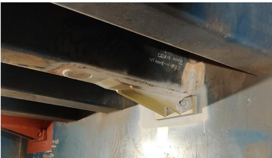
**Figure 26: Repair of a trough to cross girder connection with a 'kano'**
