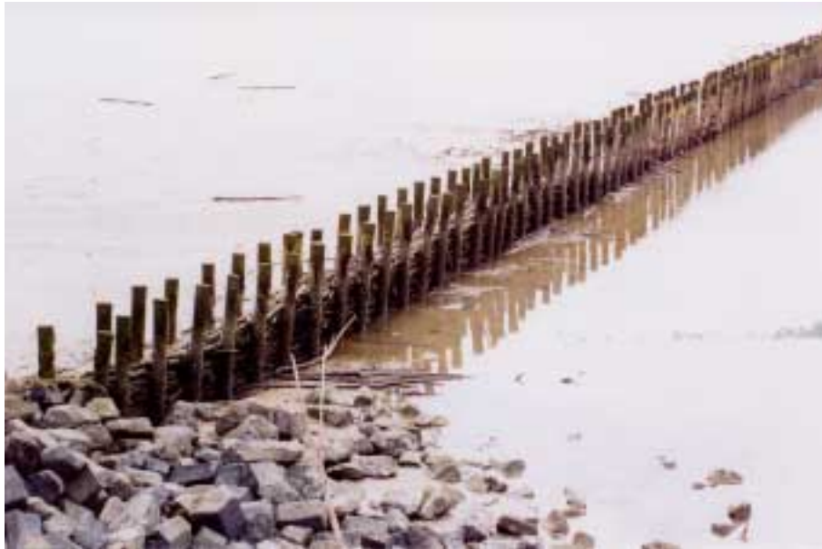
Figure 68. Accreting faggot, Holwerd, The Netherlands
