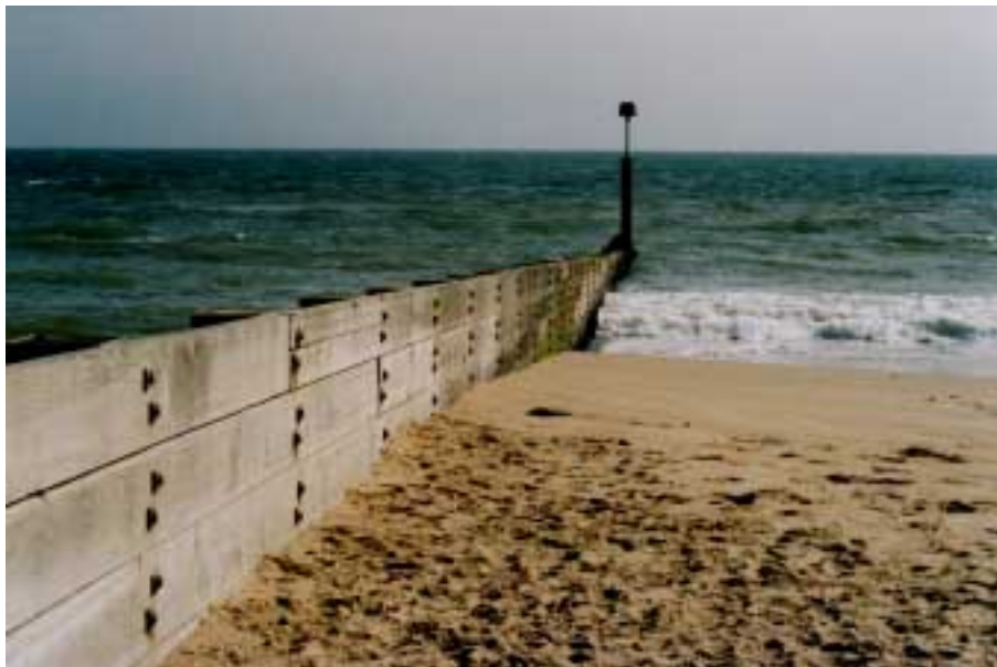
Figure 27. High quality groyne at Bournemouth
