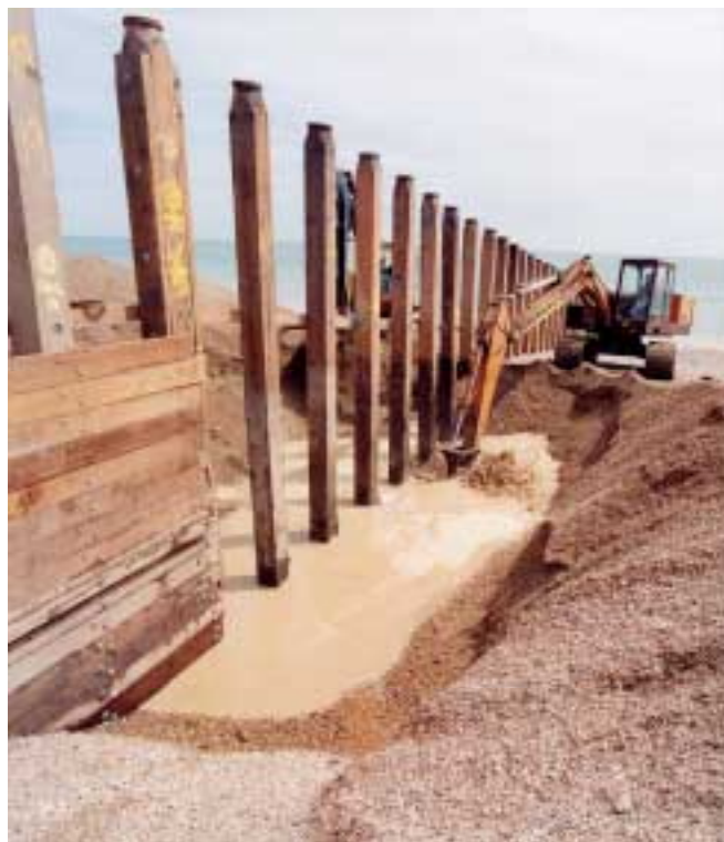
Figure 45. Excavating in order to attach planking (courtesy to Posford Haskoning)
