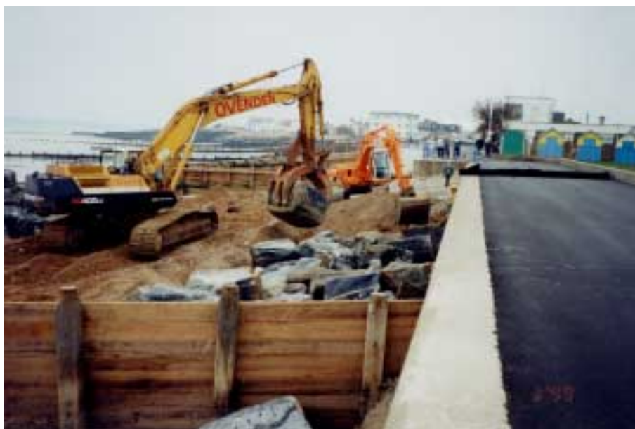
Figure 33. Groynes at Felpham with rock toe in front of seawall (courtesy to Posford Haskoning)
