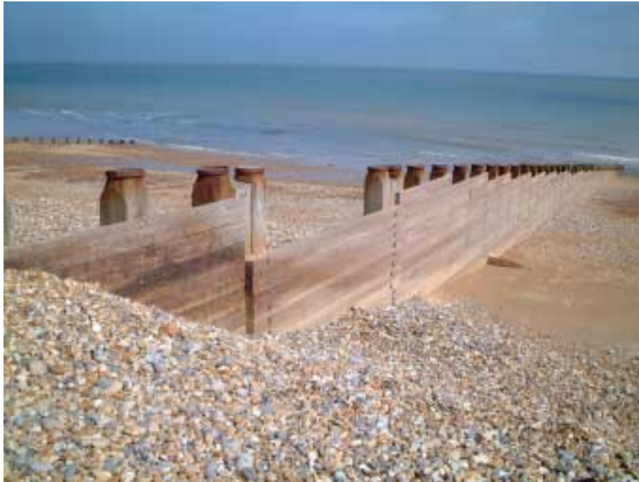
Figure 32. Groyne with plant access bay
