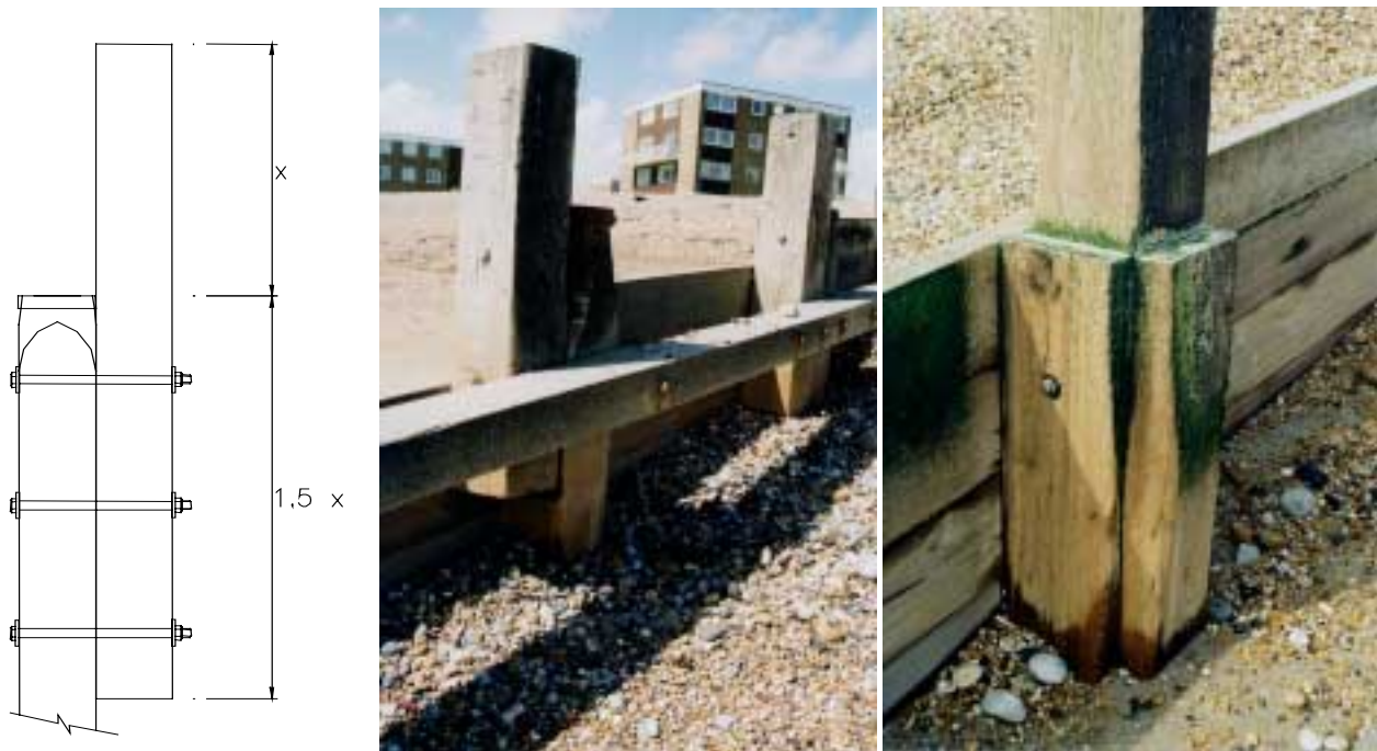
Figure 58. Pile extension Figure 59. Rubbing pieces
