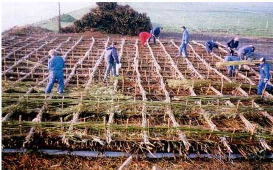
Figure 67. Construction of a fascine mattress (courtesy to DWW)
