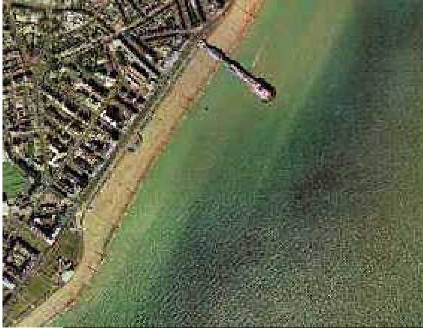
Figure 72. Aerial photograph of Eastbourne scheme (courtesy to Multimap)
