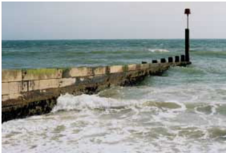
Figure 3. Conventional impermeable timber groyne (Bournemouth, UK)
