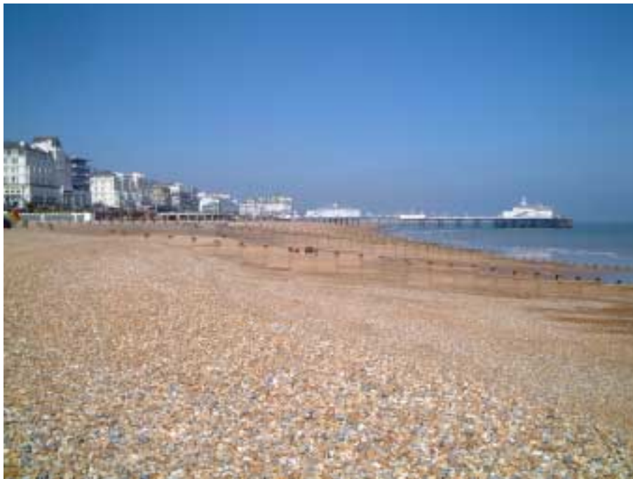
Figure 31. Overview of Eastbourne coast protection scheme
