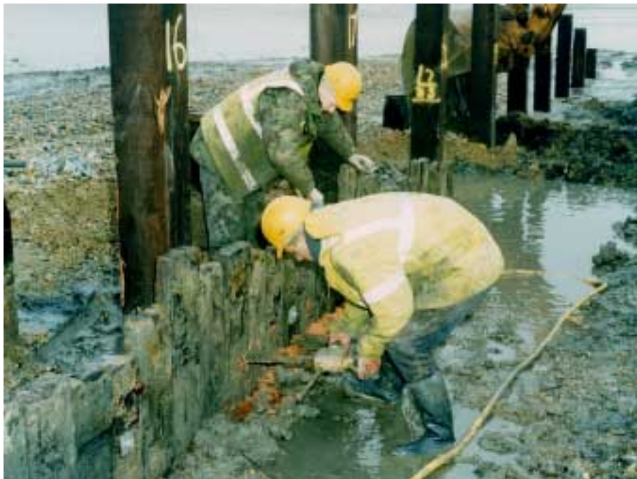
Figure 57. Attaching recycled sheeters (courtesy to Posford Haskoning)
