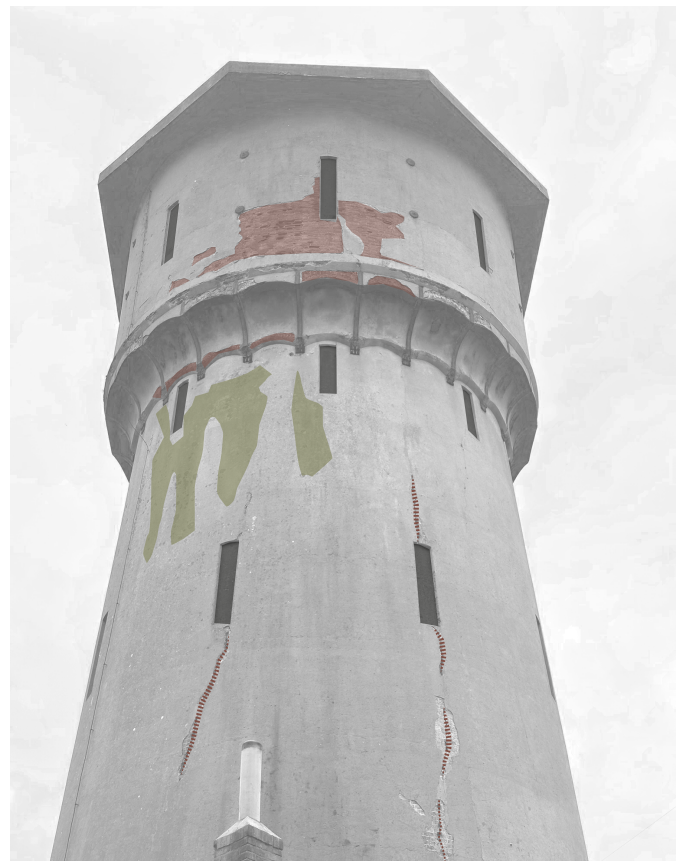
Figure 06: water tower upper part
