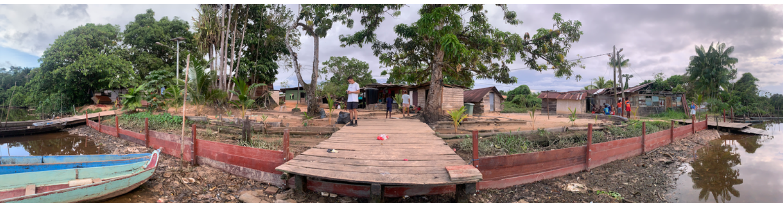
Figure 7.8: After the prototype has been build: right of the pier is the original 12 meters and left the elaborated 12 meters. Mangroves and cocospalms are planted on the soil and in the water.
