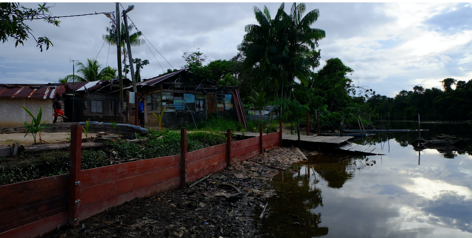
Figure 7.13 the 60cm high wooden sheet pile on the river bank further explained on the educational board at the river bank.
