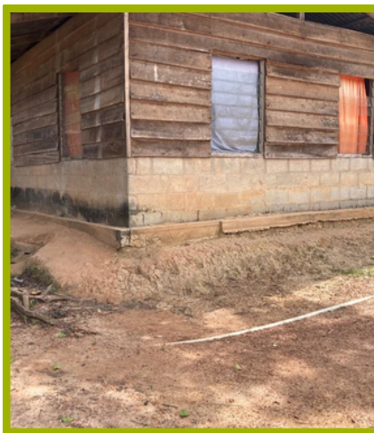
soil erosion by extended periods of heavy rainfall
