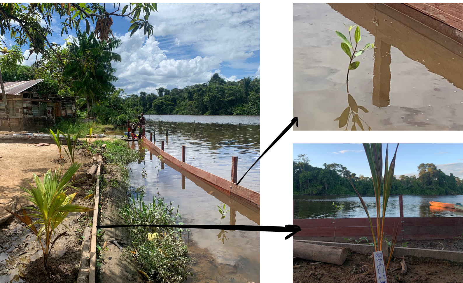
Figure 7.10: The river bank protection with cocos palm trees (on dry soil), mangroves between layers of terraces (in the water), and zoomed in into these two.
