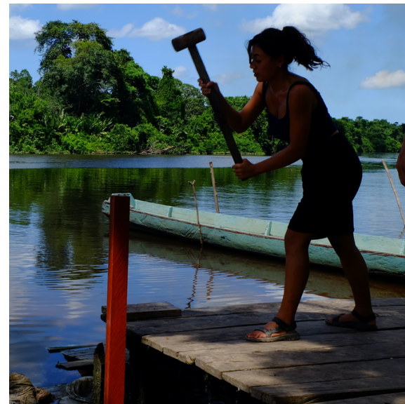
Figure 7.5: First, the holes are dug (left), after which the poles are pressed into the ground using the hand piling device (middle) or the sledgehammer (right)
