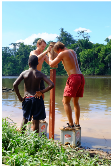
Figure 7.5: First, the holes are dug (left), after which the poles are pressed into the ground using the hand piling device (middle) or the sledgehammer (right)
