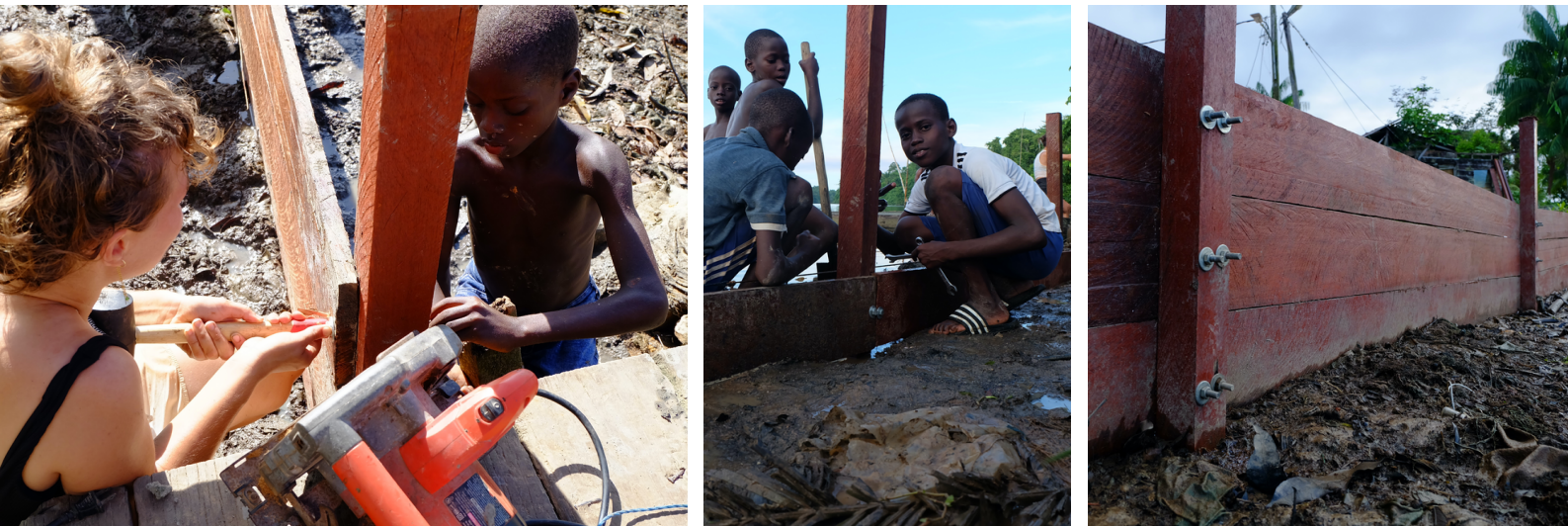
Figure 7.6: The planks are sawn at the exact length using the circular saw and then attached to the poles using a drill and 12mm nut bolts
