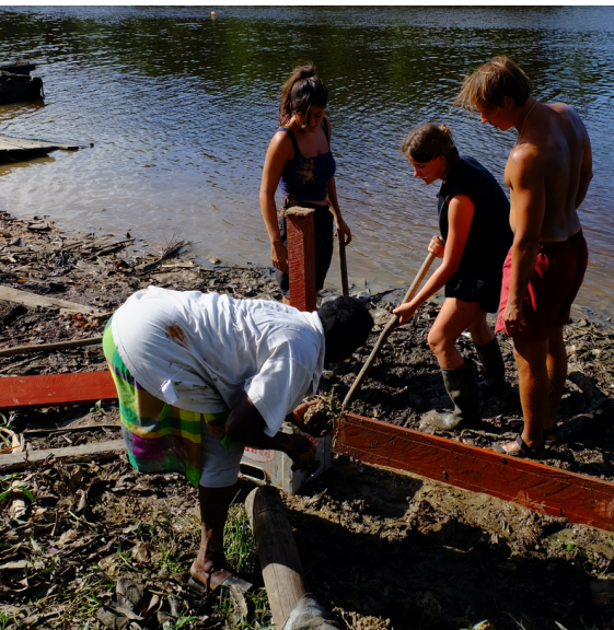
Figure 7.5: First, the holes are dug (left), after which the poles are pressed into the ground using the hand piling device (middle) or the sledgehammer (right)
