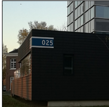
The facade of ground floor is close
