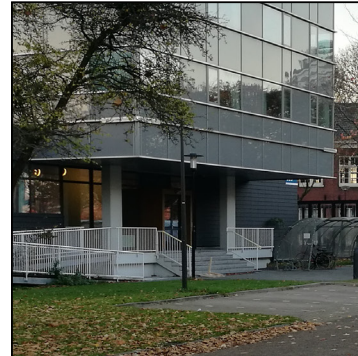
Exposure of structure on ground floor
