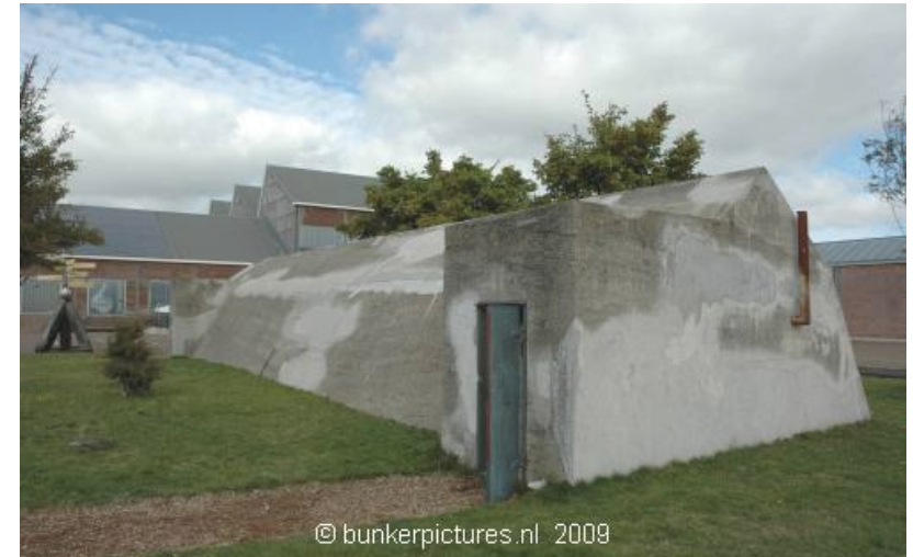
figure 5 - 19 raid shelter, with central heating and a pit-coal storage source: Forten, bunkers in Den Helder.
