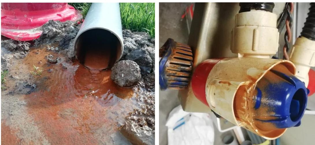
Figure 28: Oxidised iron in outflow pipe and on pump
