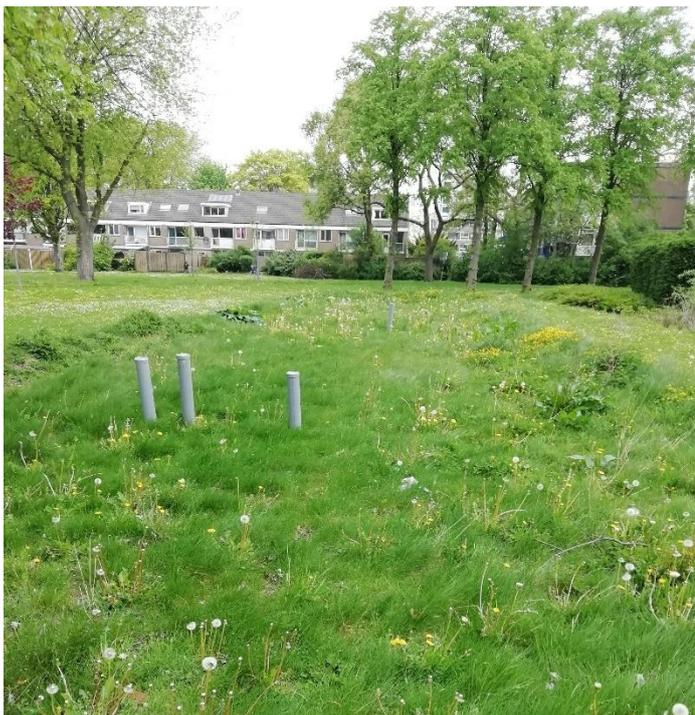
Figure 50: Picture bioswale 7, dike separating the swale from the surrounding area
