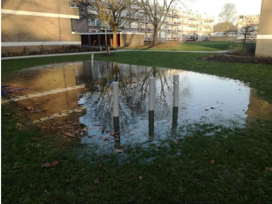
Figure 14: Picture bioswale D after filling
