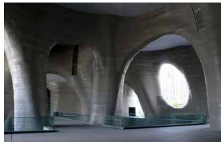
(b) Freeform support structures.
