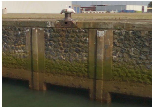
Figure 10: Bollards and granite columns along the quay wall at the portside of Pier 1 (Port of Rotterdam)
