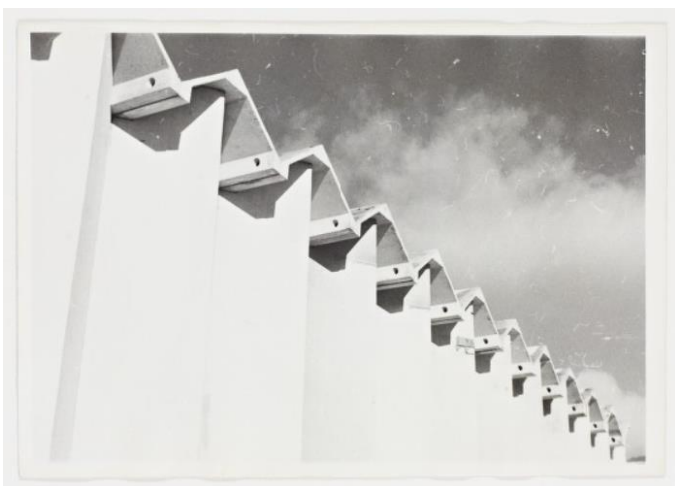
Fig. 20 Conference building, wall-roof connection
