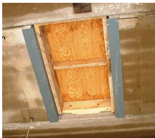
Figure 30: Bottom view of closed recess in hollow-core slab by using plywood panel. Source: Havel [44].
