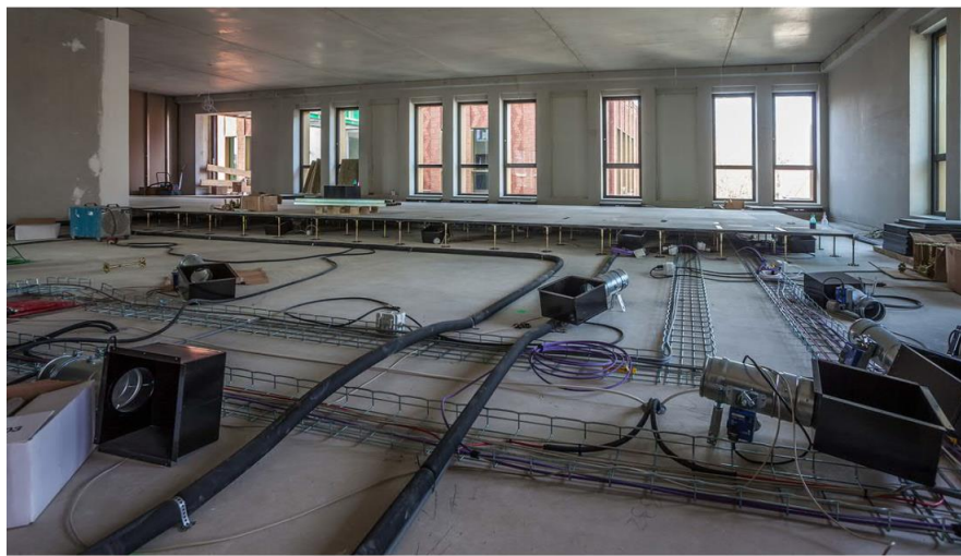
Figure 29: Solution of elevated floor to separate installations from structure. Source: ABT [2].
