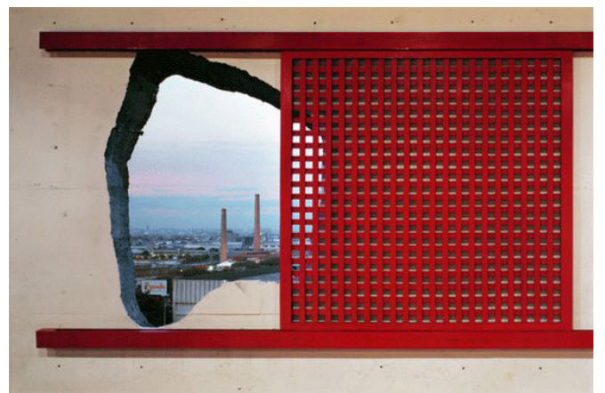
openings in the sports tower
