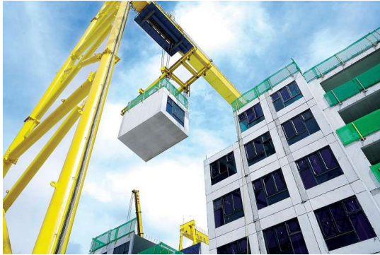
Figure 1.1: PPVC construction in Singapore [5]
