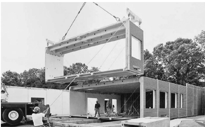
Figure 2.9: Concrete module for school building [30]
