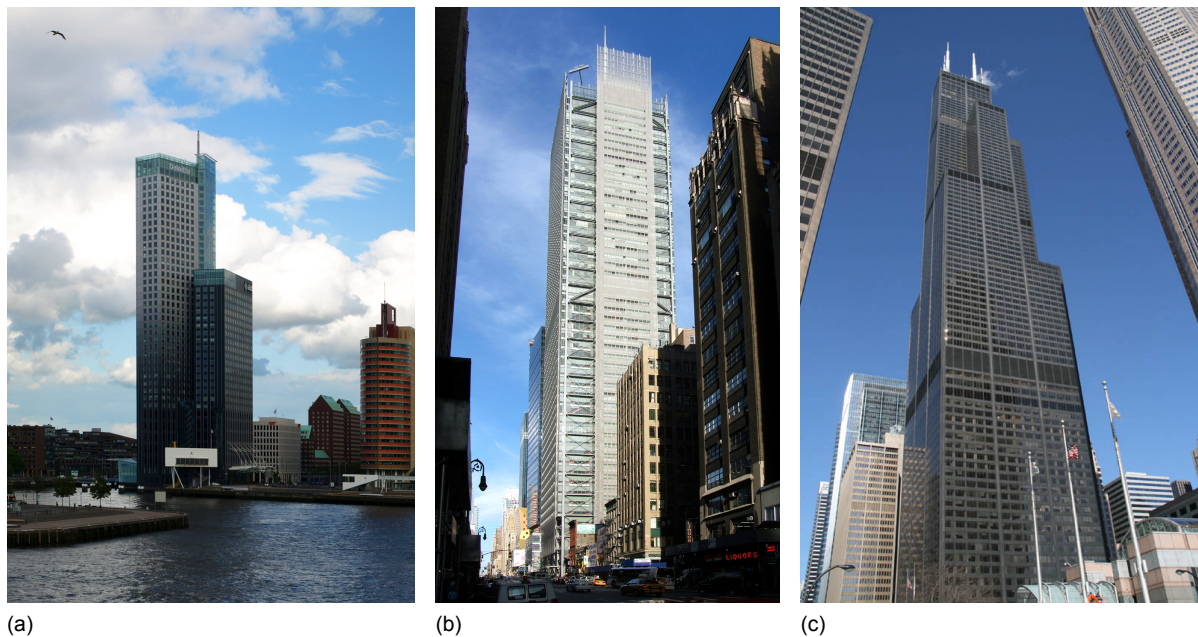
Figure 2.4: Maastoren in Rotterdam (2.4a), New York Times Tower (2.4b) and Willis Tower in Chicago (2.4c) [26]
