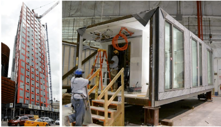
Figure 5.8: Module in 461 Dean Street Building [7]
