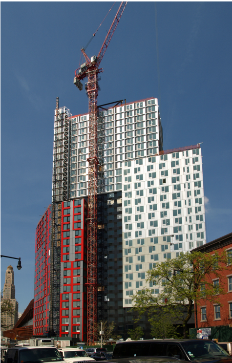
Figure 2.11: 461 Dean Street, New York during construction [26]
