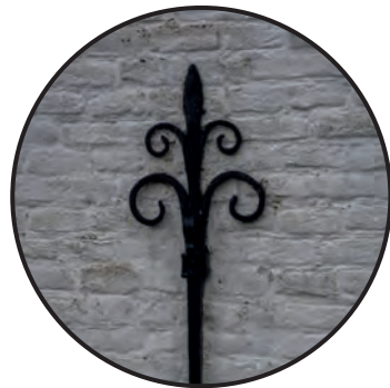
Wrought iron wall anchors
