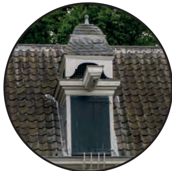
Wooden lifting hatch with slated roof
