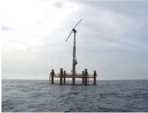
Figure 1.1: World's first floating wind turbine 6 .
