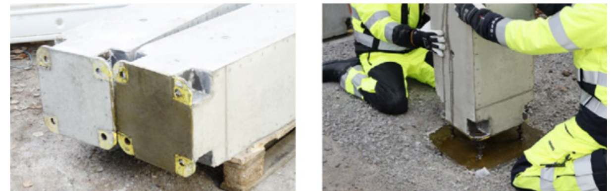
Figure 17: Demountable Concrete column detail | Source: Yrjölä (2022)
