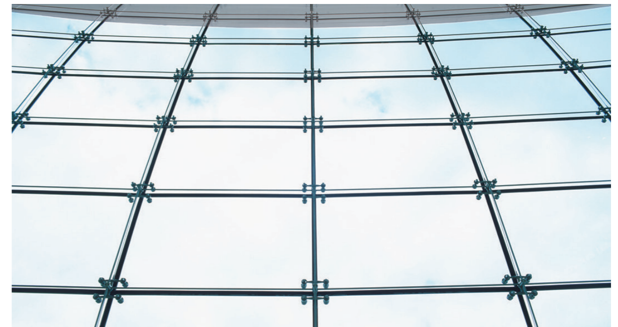
Figure 5: Bolted Connections, Seattle-Tacoma International Airport | Source: novumstructures.com
