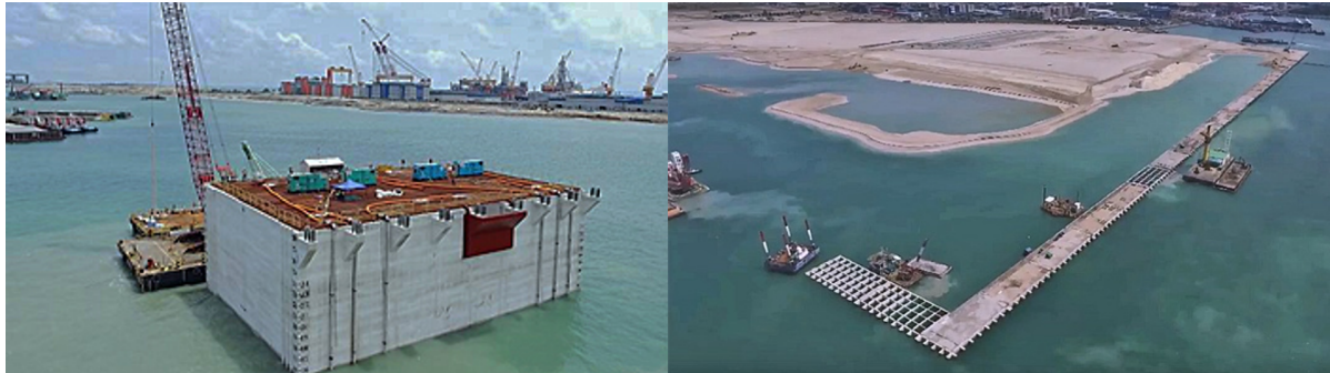
Figure 2.9: Tuas Port, Singapore. Left: towing of a caisson. Right: outline of caissons. Images: (Royal Boskalis, 2025).
