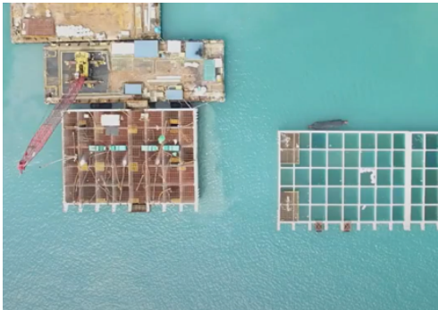
(b) Caissons placed for the Tuas Port project in Singapore, showing the cell structure (Singapore, 2019).
