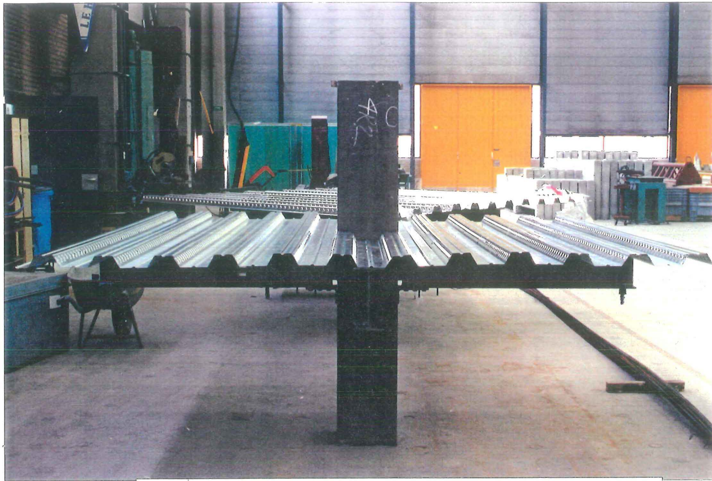
Photo 4-7 : Placement of steel decks on specimen in CHS
