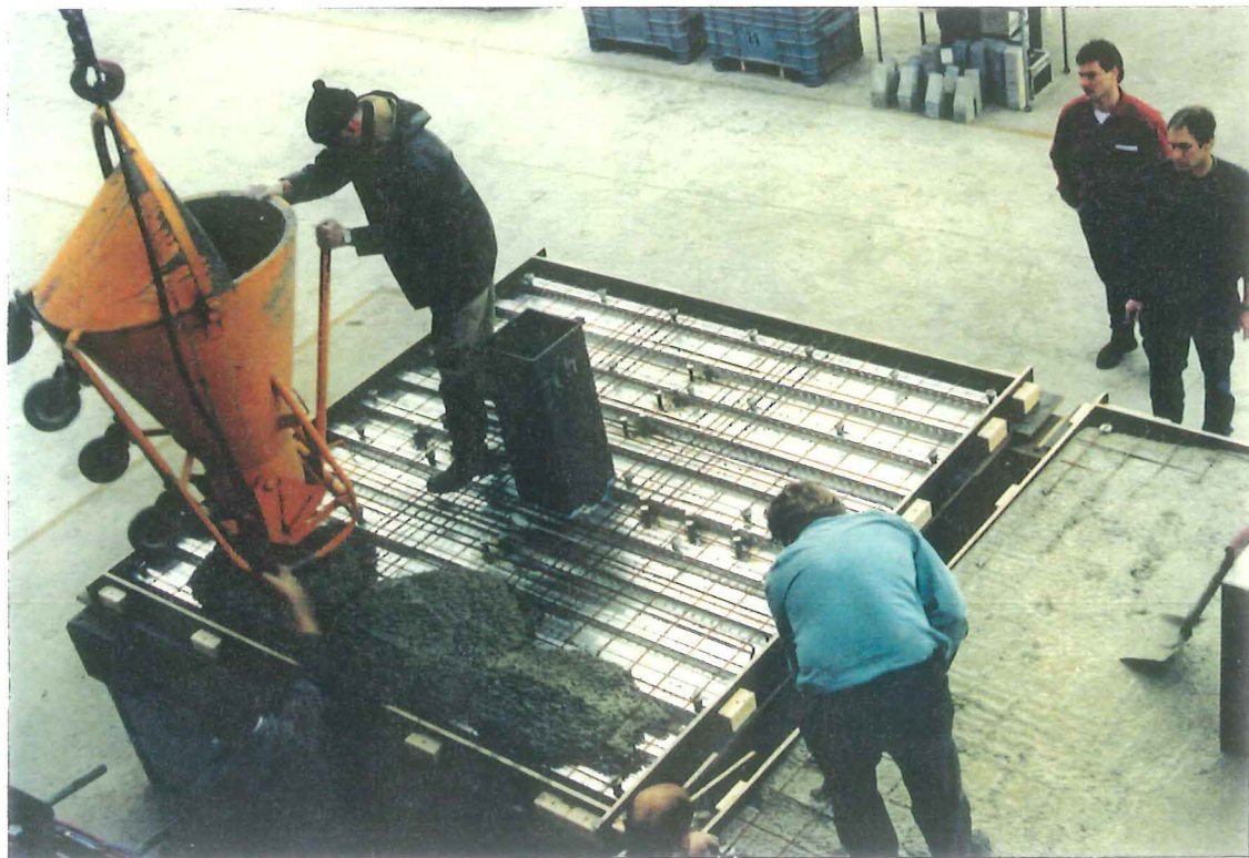
Photo 4-10 : Concreting
