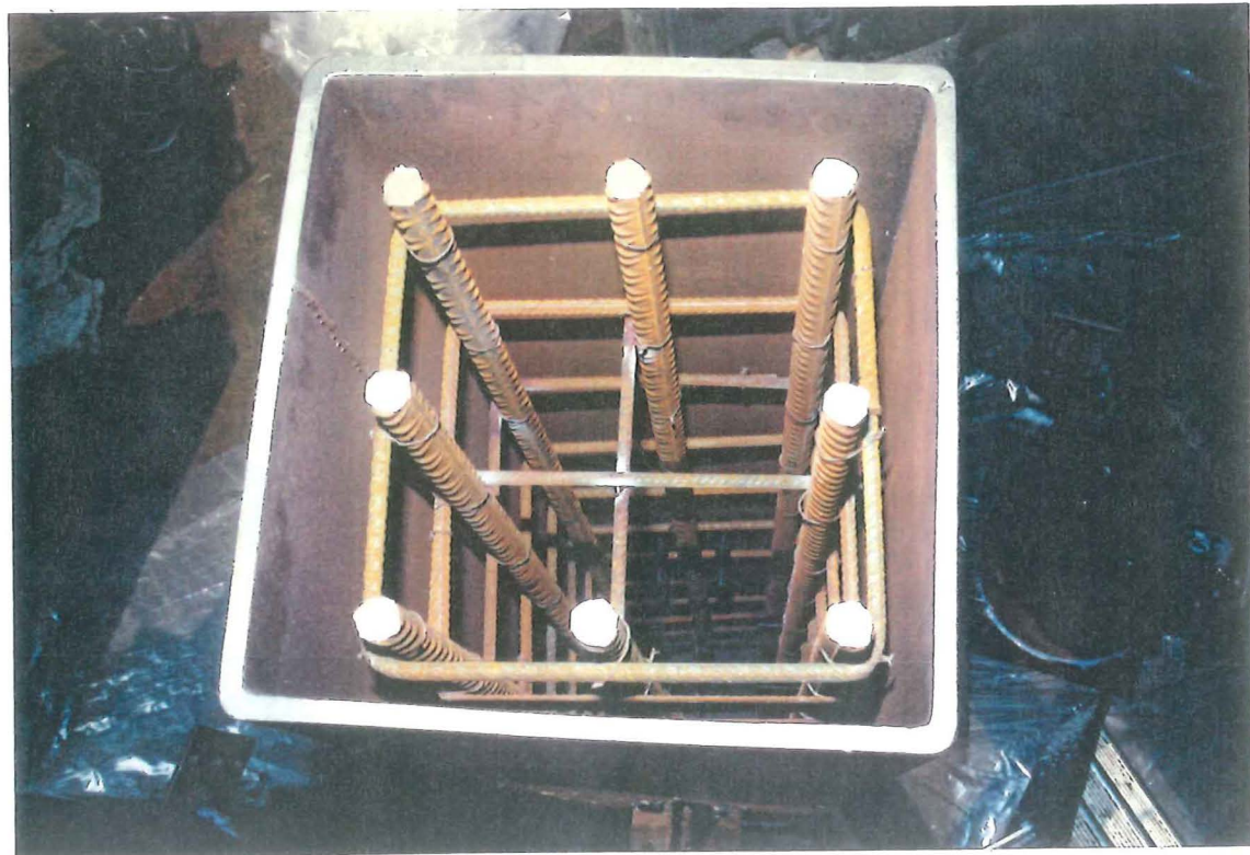
Photo 4-4 : Reinforcement arrangement inside RHS columns
