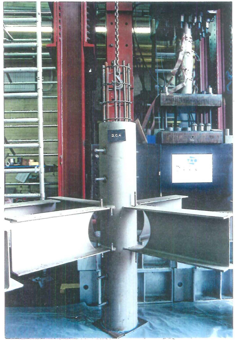
Photo 4-2 : Placement of reinforcement cages of typical CHS columns
