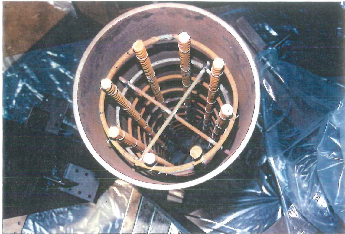
Photo 4-3 : Reinforcement arrangement inside CHS columns
