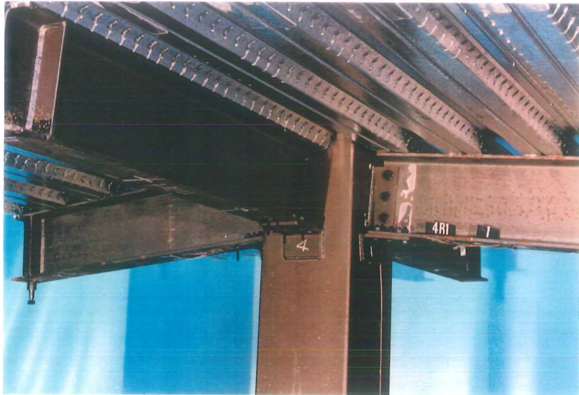
Photo 7-30 : Specimen 4R1 after failure
