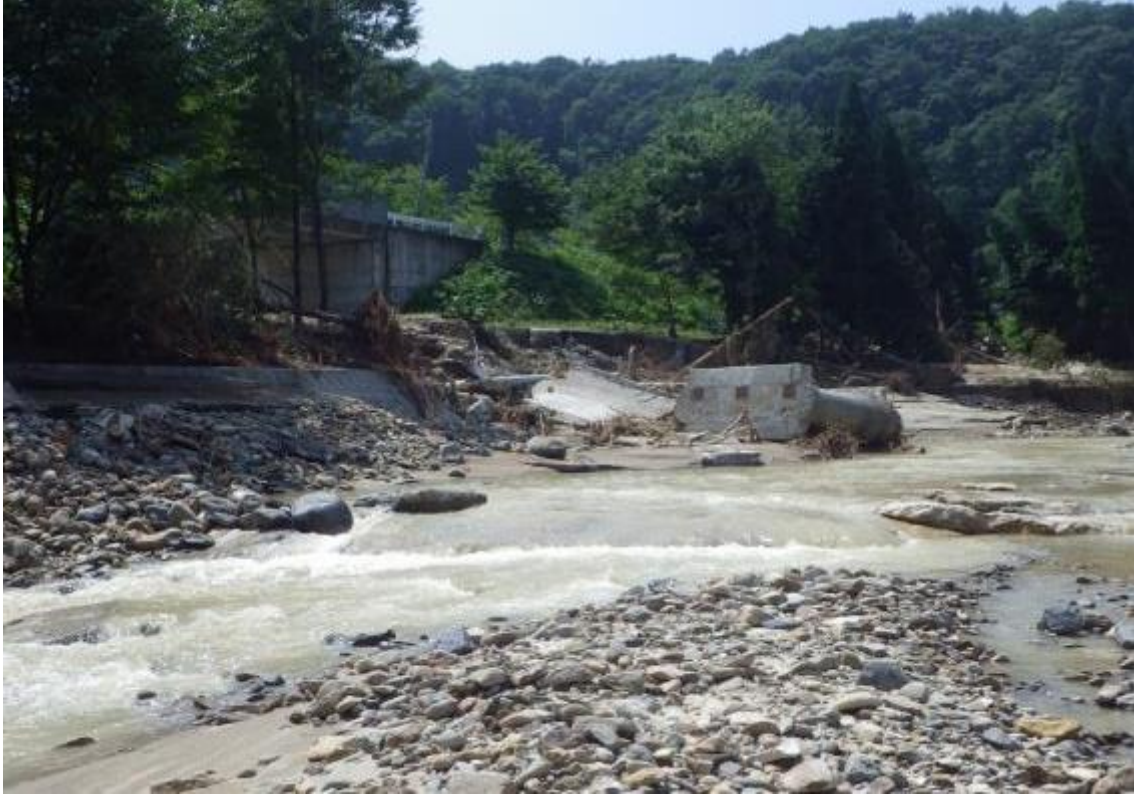
Figure 4: Photo of the collapsed southern pier (taken by J.D. Bricker, 2013)
