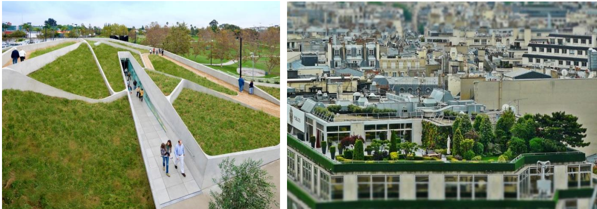
Figure 28. Extensive (left) and intensive (right) green roof (Resources: 2030 PALETTE and Skyluxe)
