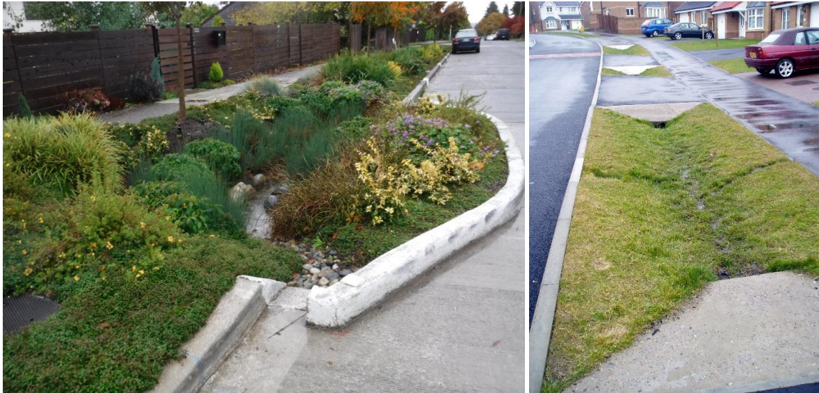
Figure 27. Bioretention cell (left) and Vegetated Swales (right) (Resources: NACTO and Susdrain)
