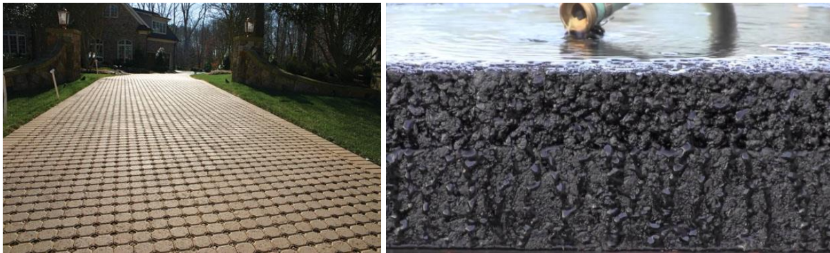
Figure 29. Permeable interlocking pavers (left) and Porous asphalt (right) (Resources: MASONRY DESIGN and NCAT Auburn University)
