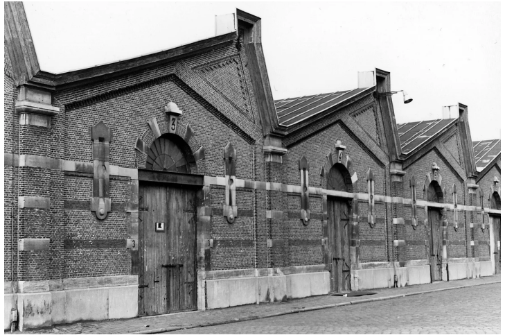
Montevideo warehouse in Antwerp. View from the outside.
