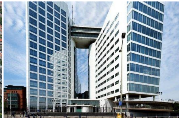
Figure 19 Front view of Haagse Arc
