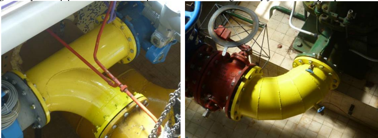
Figure 2. New pipe elements in the discharge pip of the pump house
