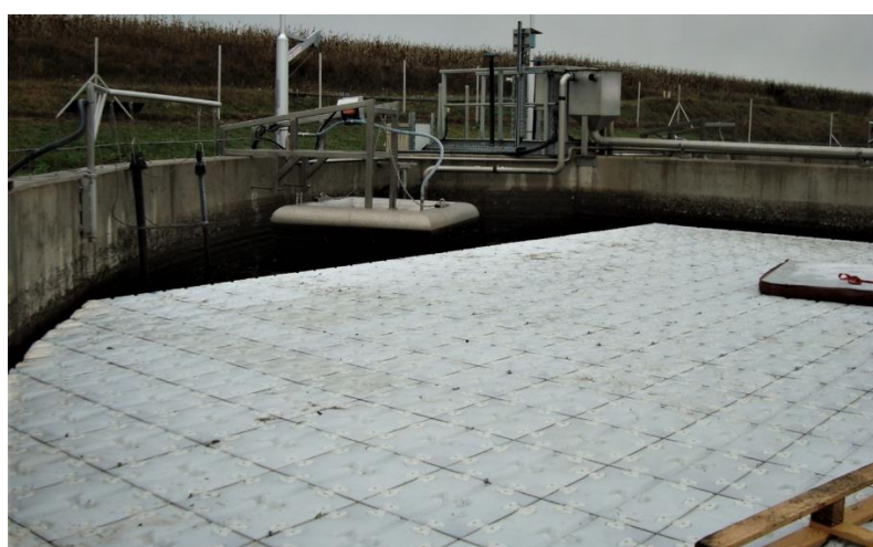
Figure 3. Seal covering the experimental system
