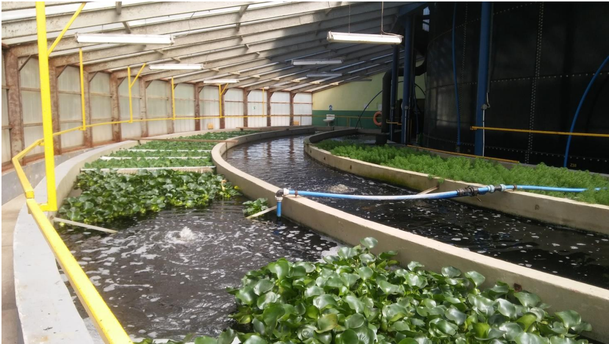
Figure 1. Hydroponic lagoon in a wastewater treatment plant in Paczków
