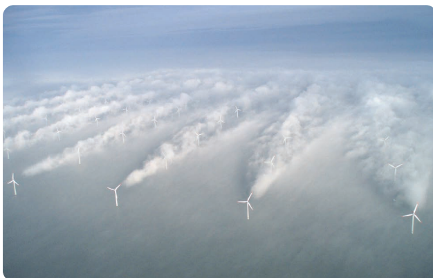
FIGURE 1 A visualization of wind turbine wakes for the Horns Rev wind farm. Atmospheric conditions were such that water vapor condensed due to the pressure change behind the wind turbines resulting in visible wakes. (Source: Image courtesy of Vattenfall, distributed under the CC BY-ND 2.0 license.)
