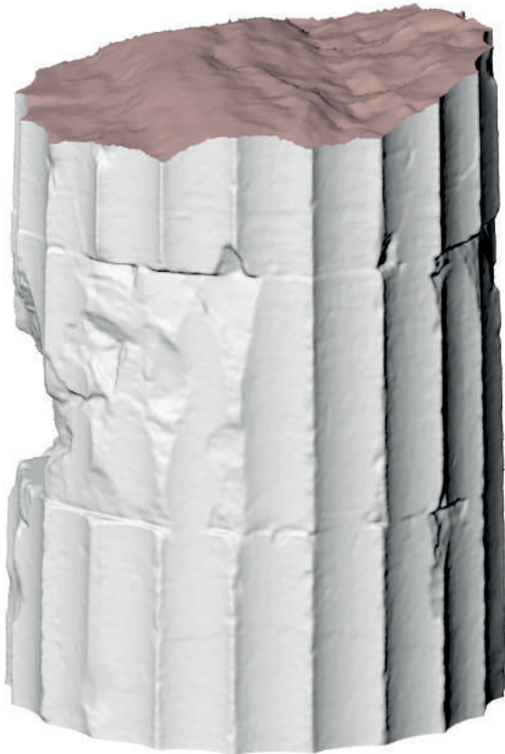
GEOMETRY OF THE LOWER PART OF THE DAMAGED COLUMN.
