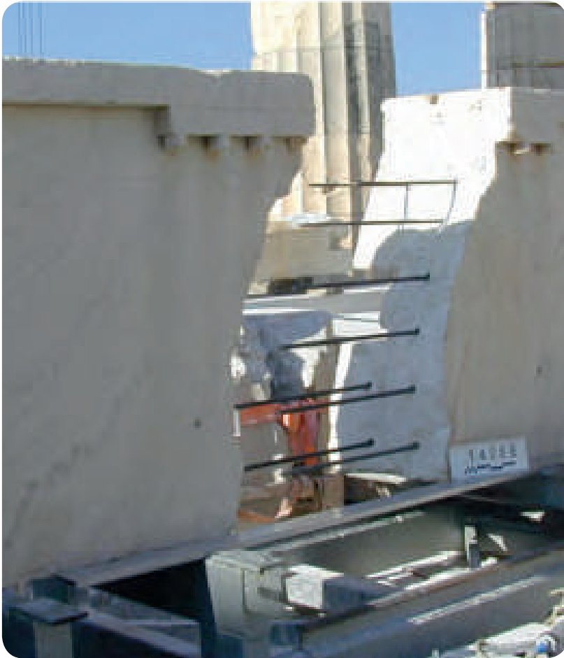
TITANIUM BARS TAKE UP THE SHEAR FORCE
