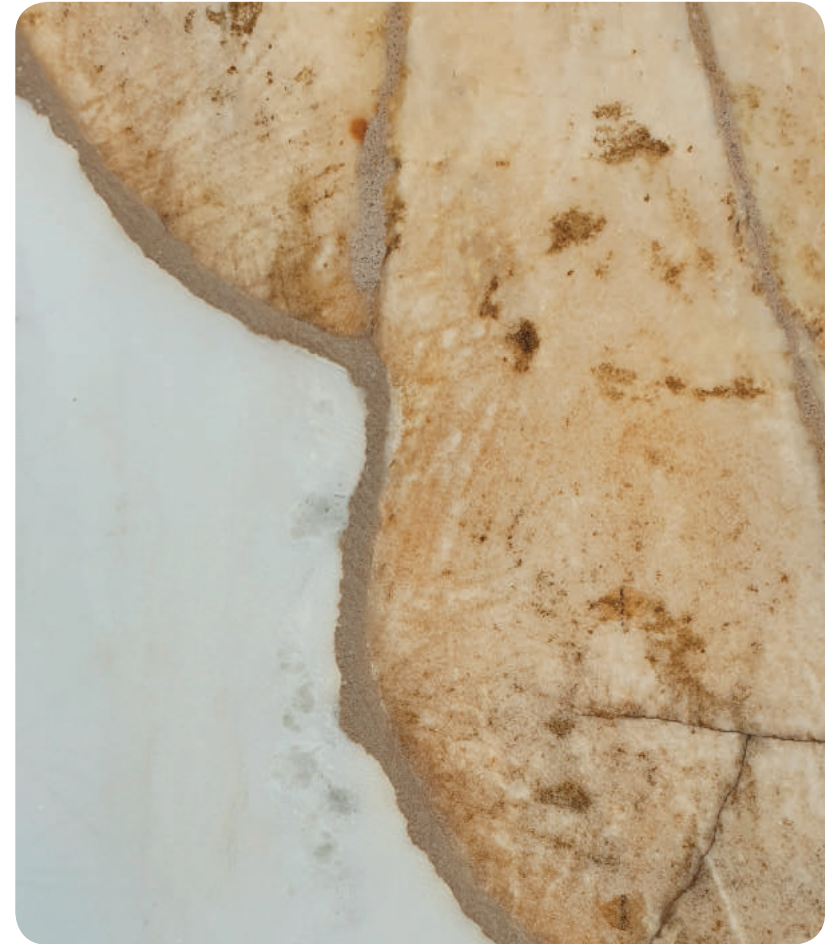
MORTAR IS USED TO SEAL GAPS, ALLOW FOR TOLERANCES AND EQUAL LOAD TRANSFER
