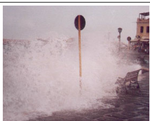
Figure 16 Overtopping at vertical harbour wall, Chania, Crete.
