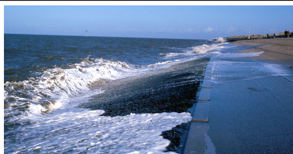
Figure 1 Run-up / overtopping on a smooth slope
