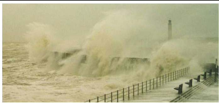
Figure 5 Wave overtopping at vertical breakwater and seawall, Margate
